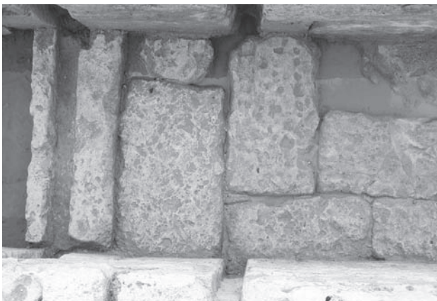
Fig. 16. Grooves and notches in the water supply channel. View from north. © MAFT
