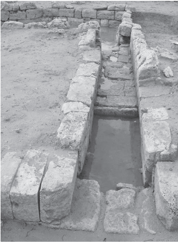
Fig. 15. Water supply channel through the eastern jetty opening into the hoop-shaped basin. View from east. © MAFT
