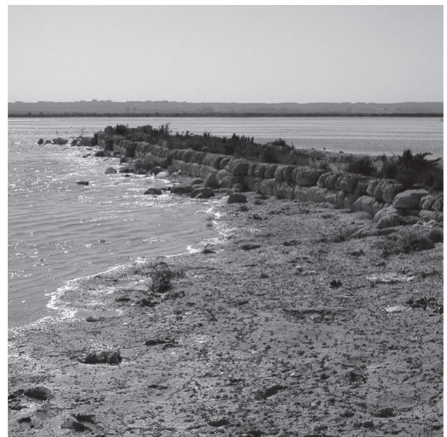
Fig. 9. The southern end of the eastern jetty. View from north. © MAFT
