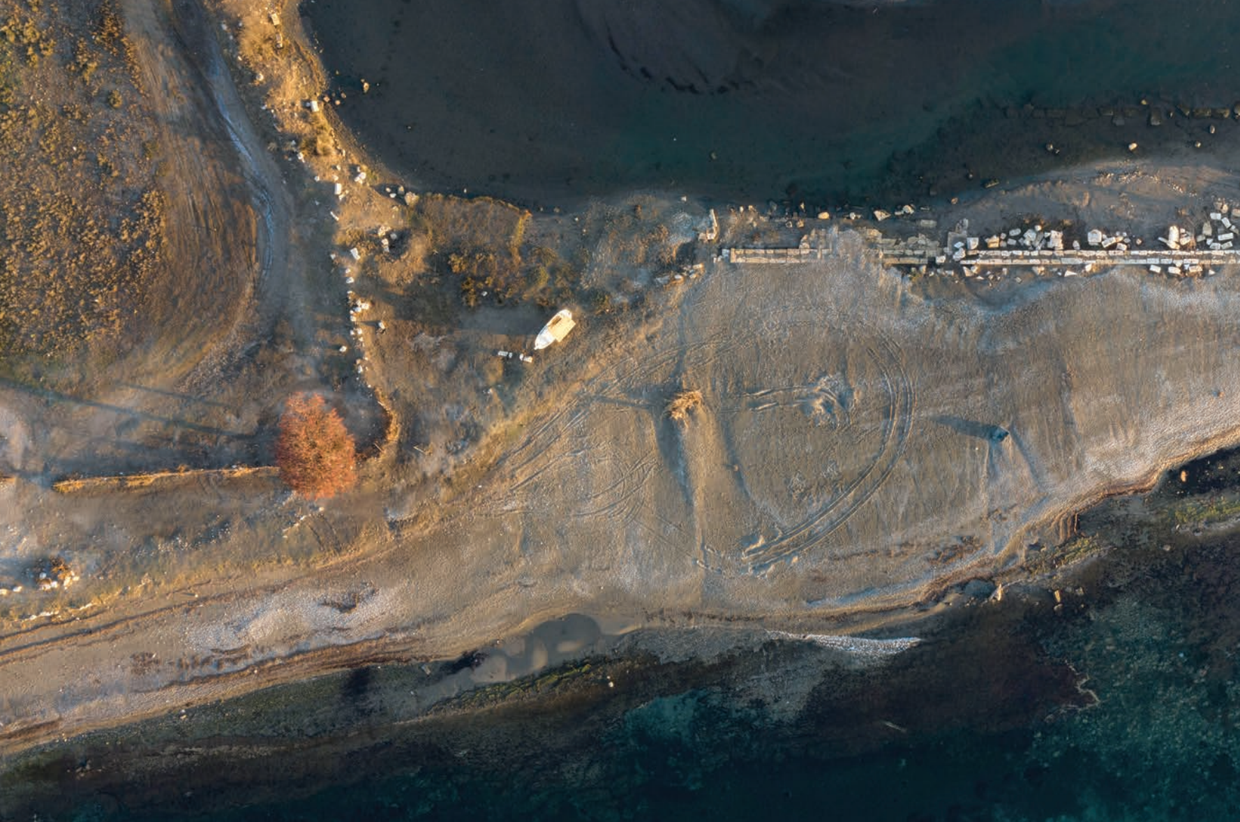
Figure 134a: Aerial photograph of the pier of the South Harbour (by C. Emden)
