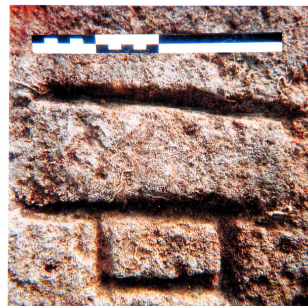
Fig. 8 - Masonry / quarrying marks on the sides of the jetty's blocks (Photo Nouredine 2004) (see also Fig. 5).
