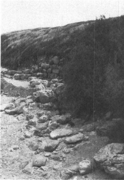
Figure 15. View of the MB II sea wall at Love Bay, Dor, looking NE.
