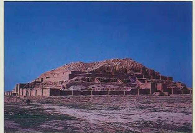
Above The construction of the ziggurat at Al-Untash-Napirisha was most unusual. The first stage of the plan was to construct a large square building about 100 m long with a central courtyard. At a later stage the central courtyard was filled in and the ziggurat built inside it.
