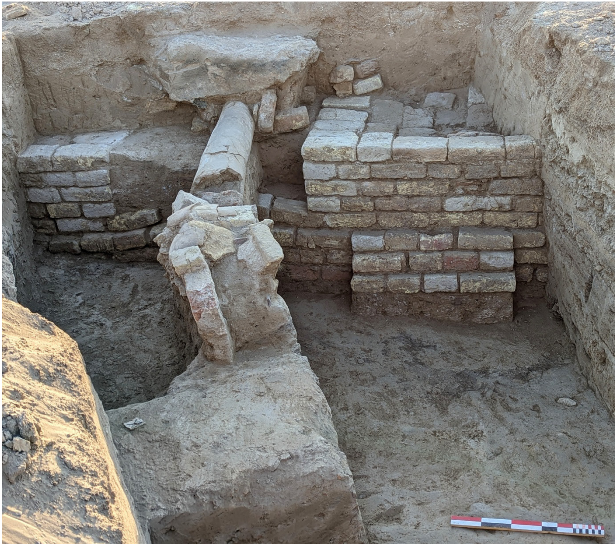
Fig. 7 – Trench H1: Pipe C132 discharging into the Grand Canal C3 through the fired brick quay, from the west (photo R. Vallet, 2023).
