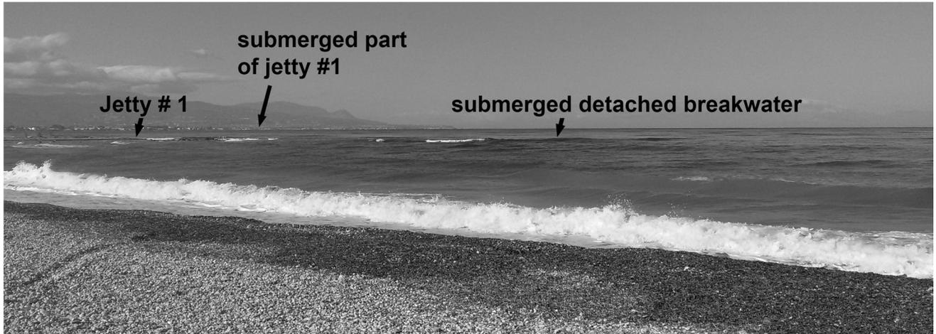
Figure 6. View of the breaking zone relatively to shore, for the T shaped submerged structure developed around jetty #1. Similar conditions are observed also for jetty #2.
