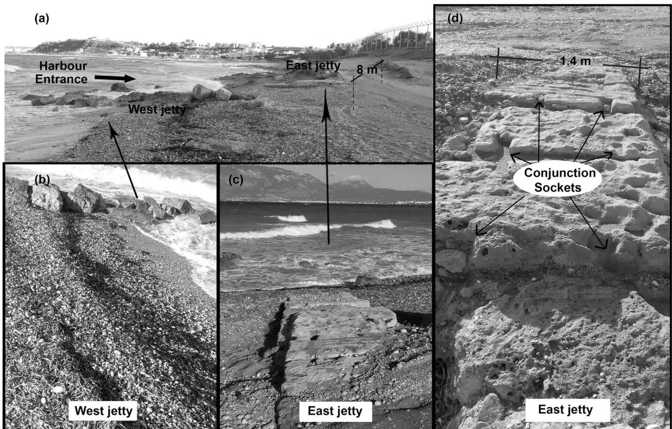
Figure 3. (a) The arrangement of the edges of the access channel, of about 8 meters wide. (b) The west jetty on the entrance of the harbour. (c) The east jetty of the entrance. (d) Interlocking of ashlar rectangular blocks with conjunctions.
