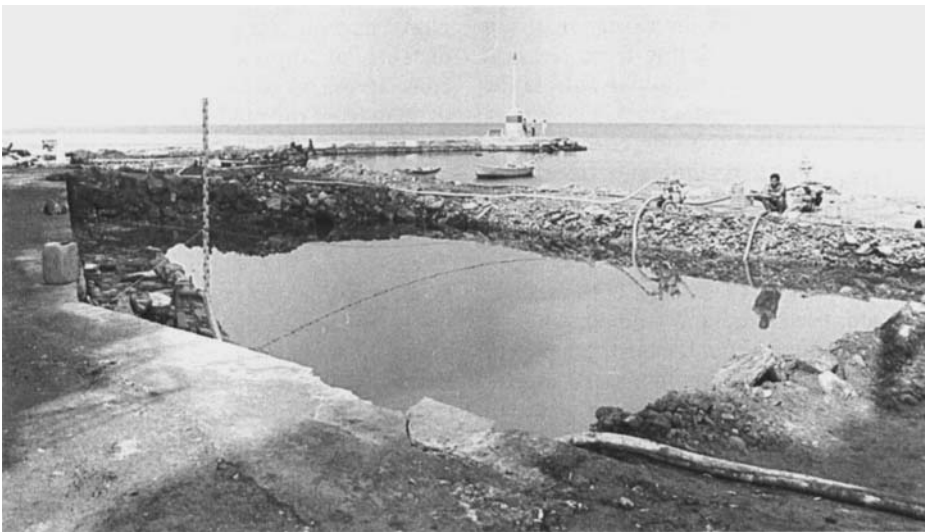
Figure 1. The port before the excavation (photograph by P. Vetzitzis).
