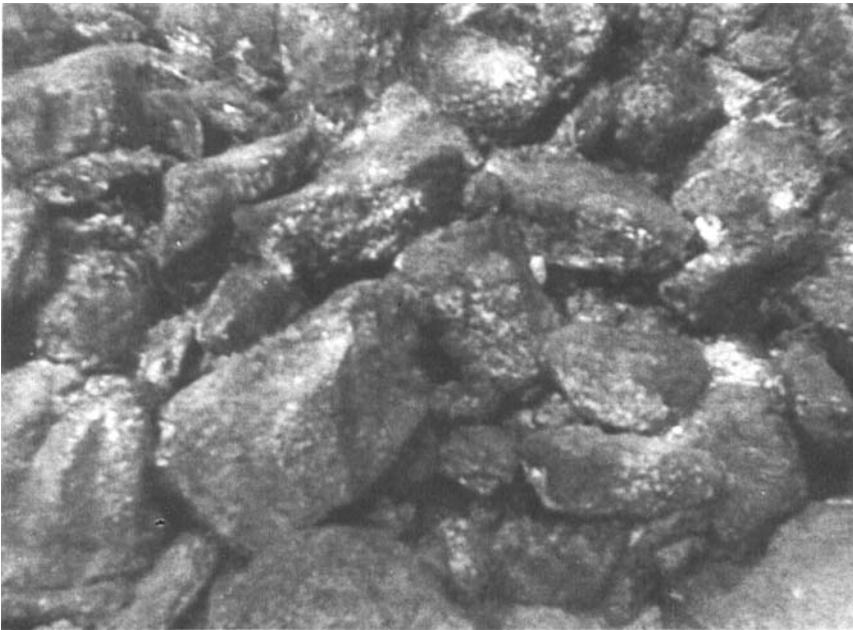
Figure 12. Northeast breakwater with medium-sized unworked stones (photograph by P. Vetzitzis).
