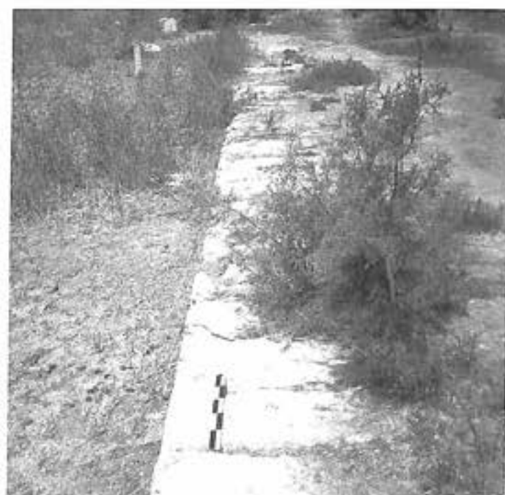
Fig. 6.66. Jetty Site 208 - header blocks.
