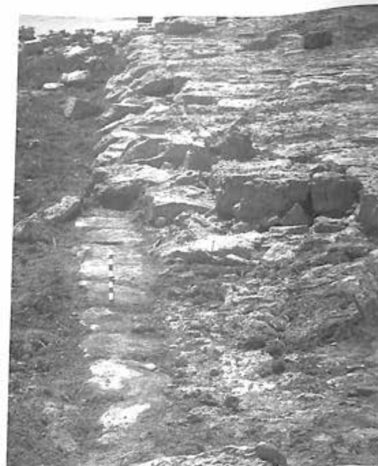
Fig. 6.69. Jetty Site 208 - header blocks.
