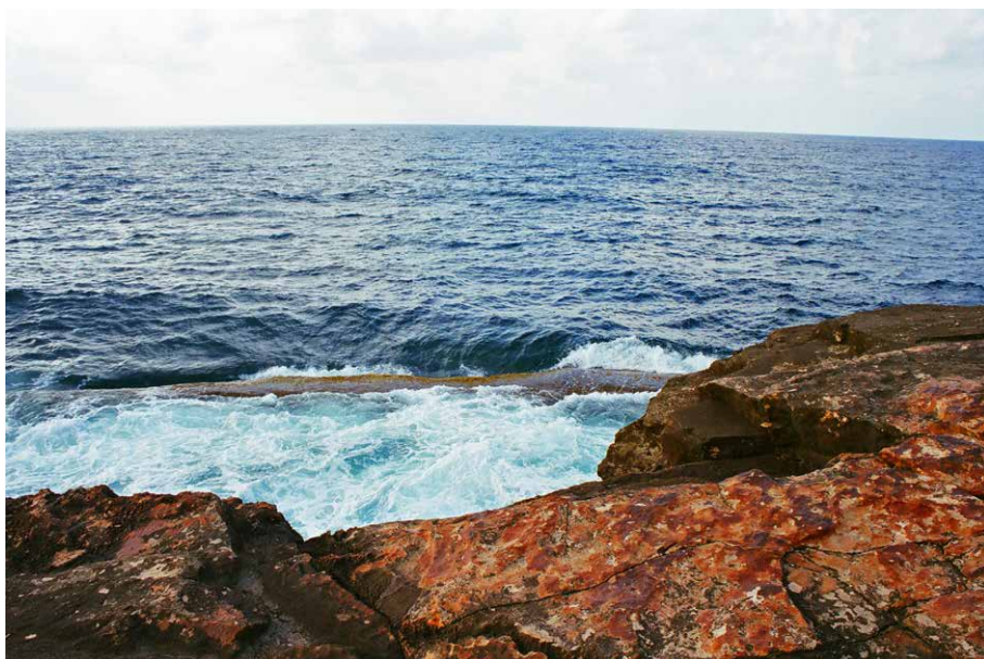
Figure 1.4. Looking down from the cliff top on the West Island at Apollonia, Libya, into the artificial wave-trap cut by divers and engineers about 2500 years ago. The ridge of rock just visible beyond the white water has been created by cutting the trough between it and the cliff. The waves break in the trough, and do not attack the cliff. The town has sunk about 2 m into the sea, so originally the wall of the wave-trap would have risen 1.5 m above still water level.
