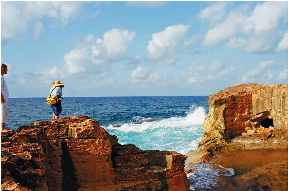
Figure 11.15. Jay Kleinberg photographs the broken wall that originally protected the West Island, both against military attack, and to prevent waves and spray washing onto the island. The ridge of the wave-trap is visible on the outside of the trough. The entrance to the storage caverns has half collapsed. Waves now wash right across the centre of the island.
