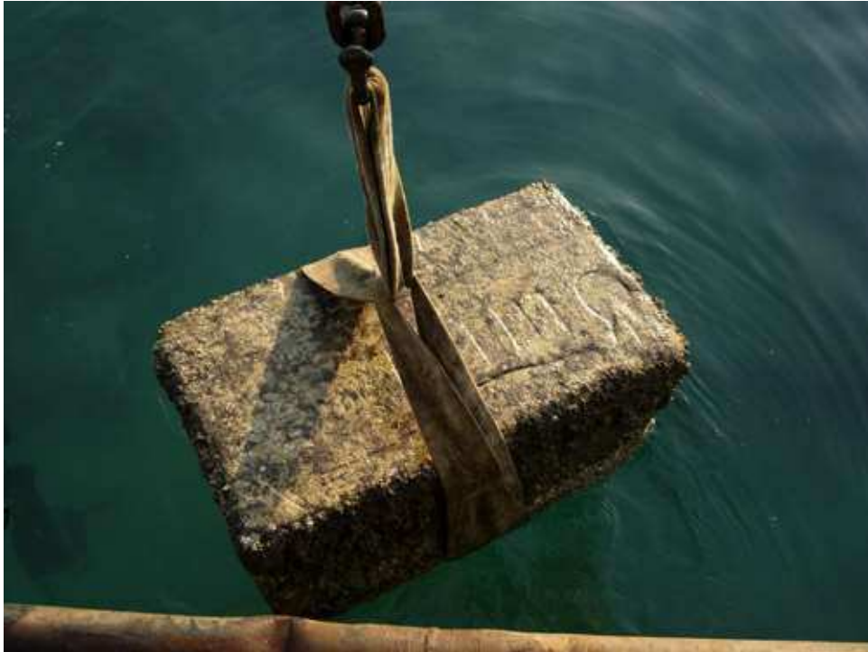
Fig. 10. Lifting a block made of quartzite inscribed with pharaonic motives using a floating crane of 50 tons lifting capacity.
