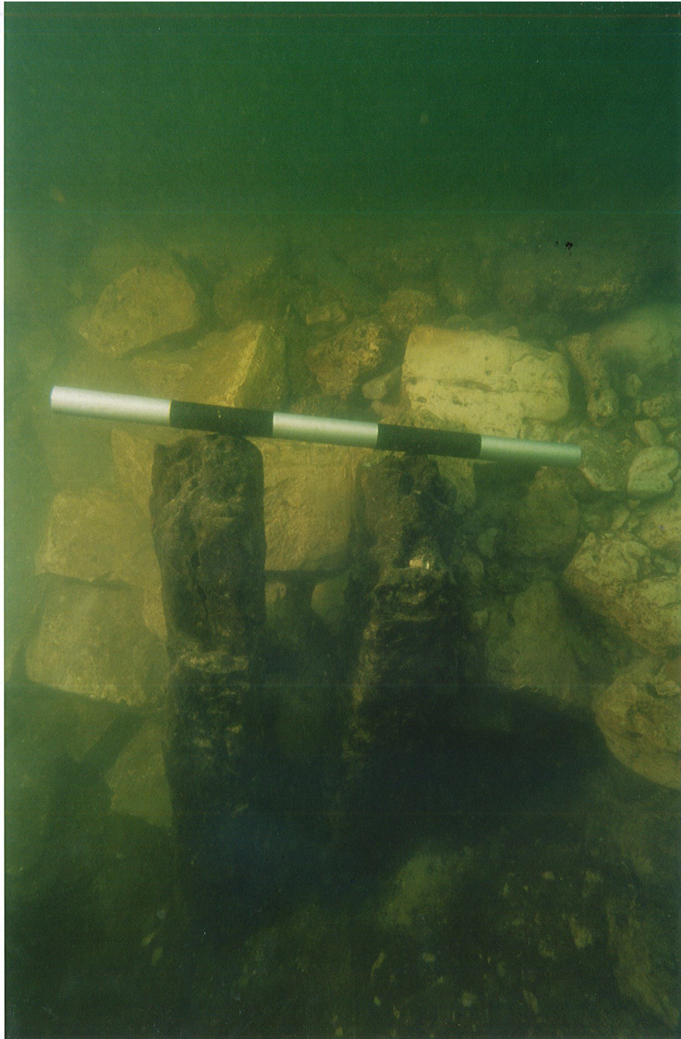
Wooden piles used to reinforce the foundations of structures built along the shores of the island of Pharos. Among the piles of small limestone blocks which they held in place, architectural fragments of ancient monuments were discovered.
