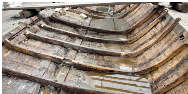
Figure 16. L-shaped floor timbers in YK 14's hull amidships, photographed during the dismantling of the hull; May 2007. (Photo M. Jones/INA)
