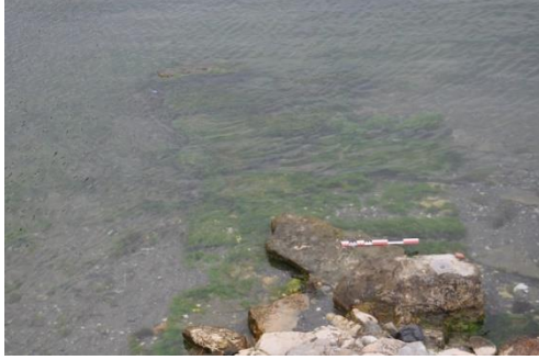
Fig. 7: Extension Part Under The Water
