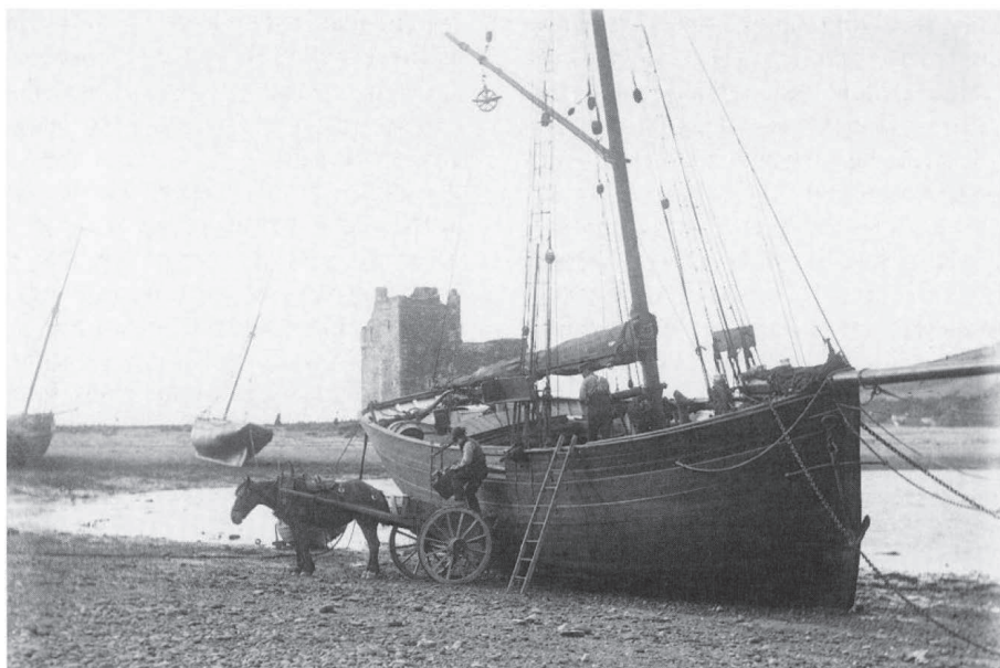
Figure 6 A nineteenth-century small coastal vessel tide beached and transferring cargo into a cart at Lochranza on the isle of Arran, Scotland; it is clear from its broadside orientation that it was not hauled out (from Houston, 'Ports in Perspective', figure 1)
