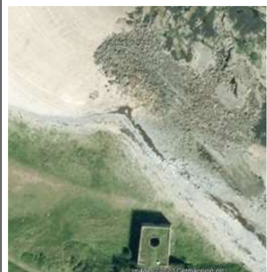
Figure 2.29 Collapsed breakwater and limekiln at Skateraw
