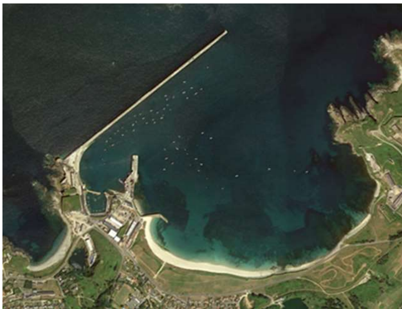
Figure 6.12 The Admiralty breakwater in 2014
