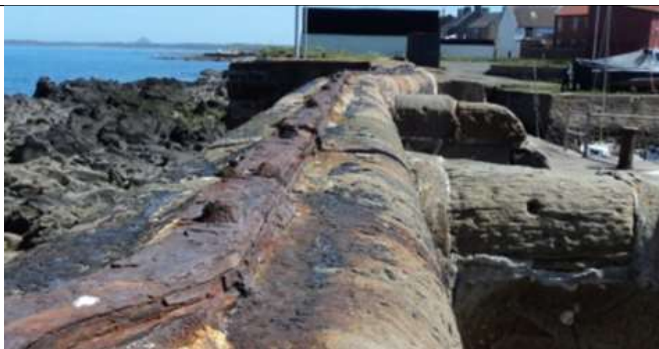
Figure D.3 Cockenzie East Breakwater
