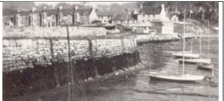
Figure D.2 Brucehaven Pier From Graham (1968)
