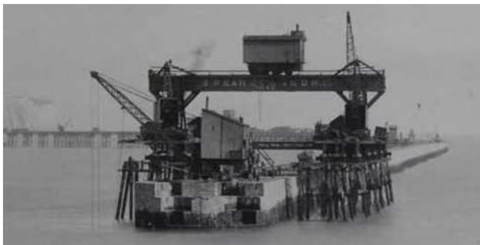
Figure 12.12 Dover - placing concrete blockwork from travelling cranes
