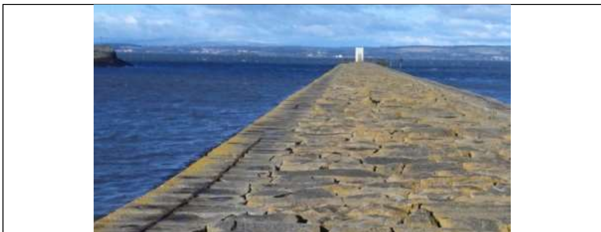
Figure D.2 Granton East Breakwater
