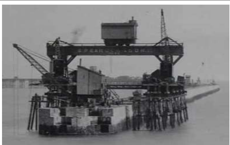
Figure 4.5 Dover - placing blockwork from travelling cranes
