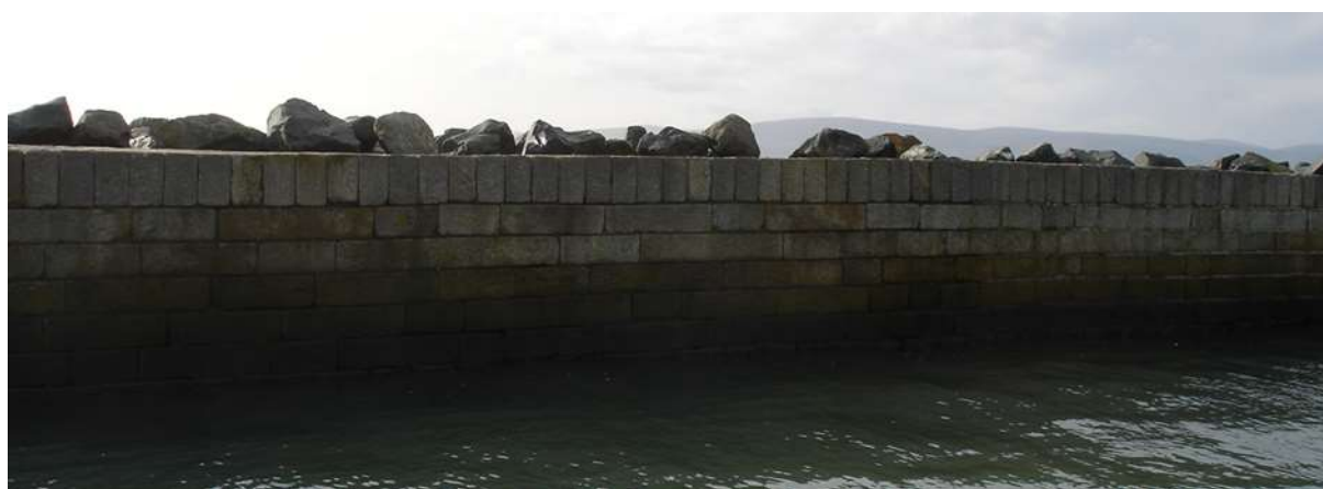
Figure 2.4 Inner face of Dublin Great South Wall
