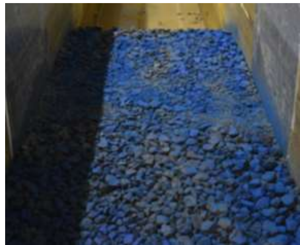
Figure 7.5 Rubble mound platform before wall construction
