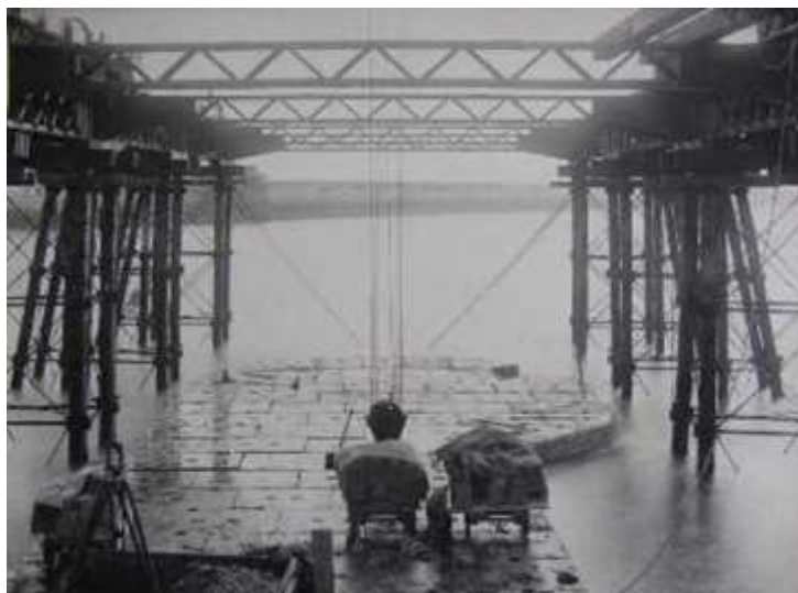
Figure 12.11 Dover - placing concrete blockwork from travelling cranes
