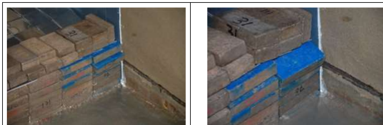
Figure 7.28 Onset of damage during Tests 138 and 139
