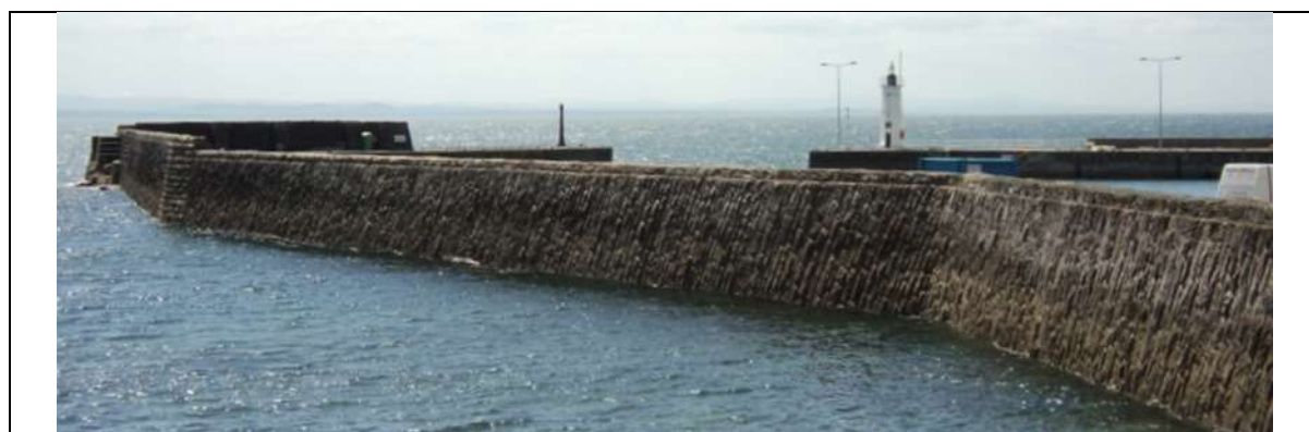
Figure D.1 Anstruther main (East) breakwater, July 2013
