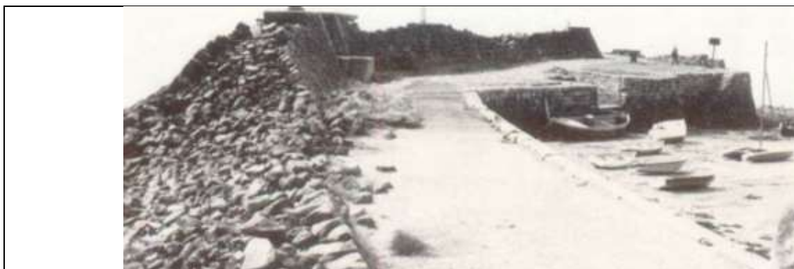
Figure D.7 Pettycur breakwater, damaged crown wall
