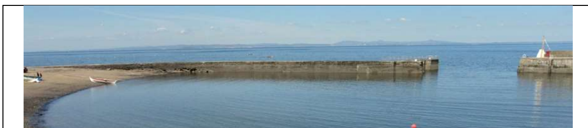
Figure D.8 Port Seton, July 2013
