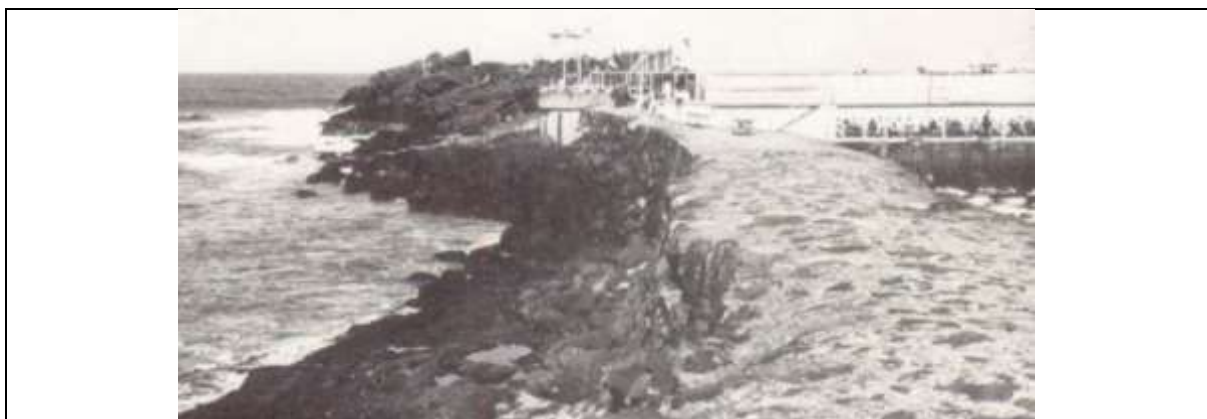
Figure D.6 North Berwick breakwater
