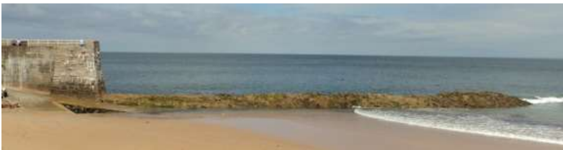
Figure 2.32 Failure at Greve du Lecq, Jersey, 1884
