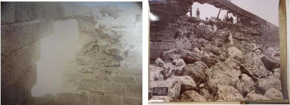
Figure 11 Breach in the parapet of the breakwater, November 1893
