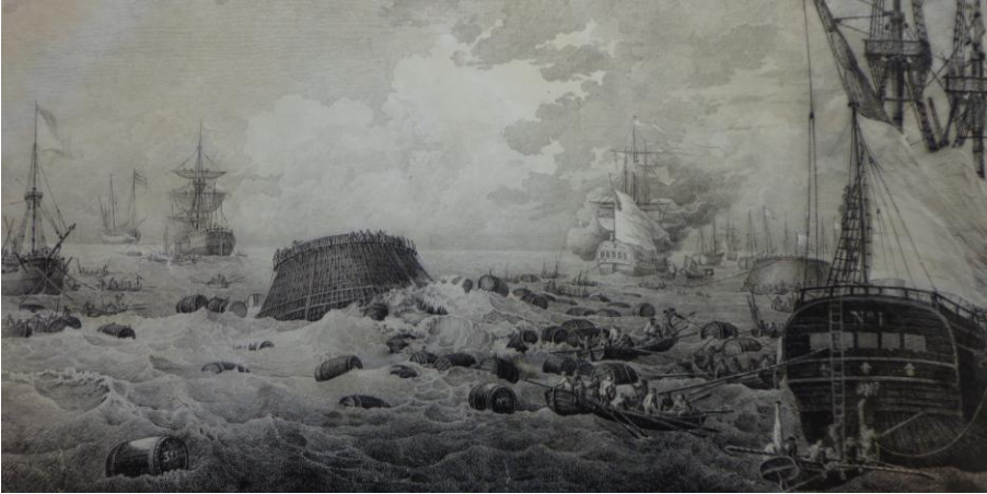
Figure 4 Sinking a cone by releasing the flotation barrels
