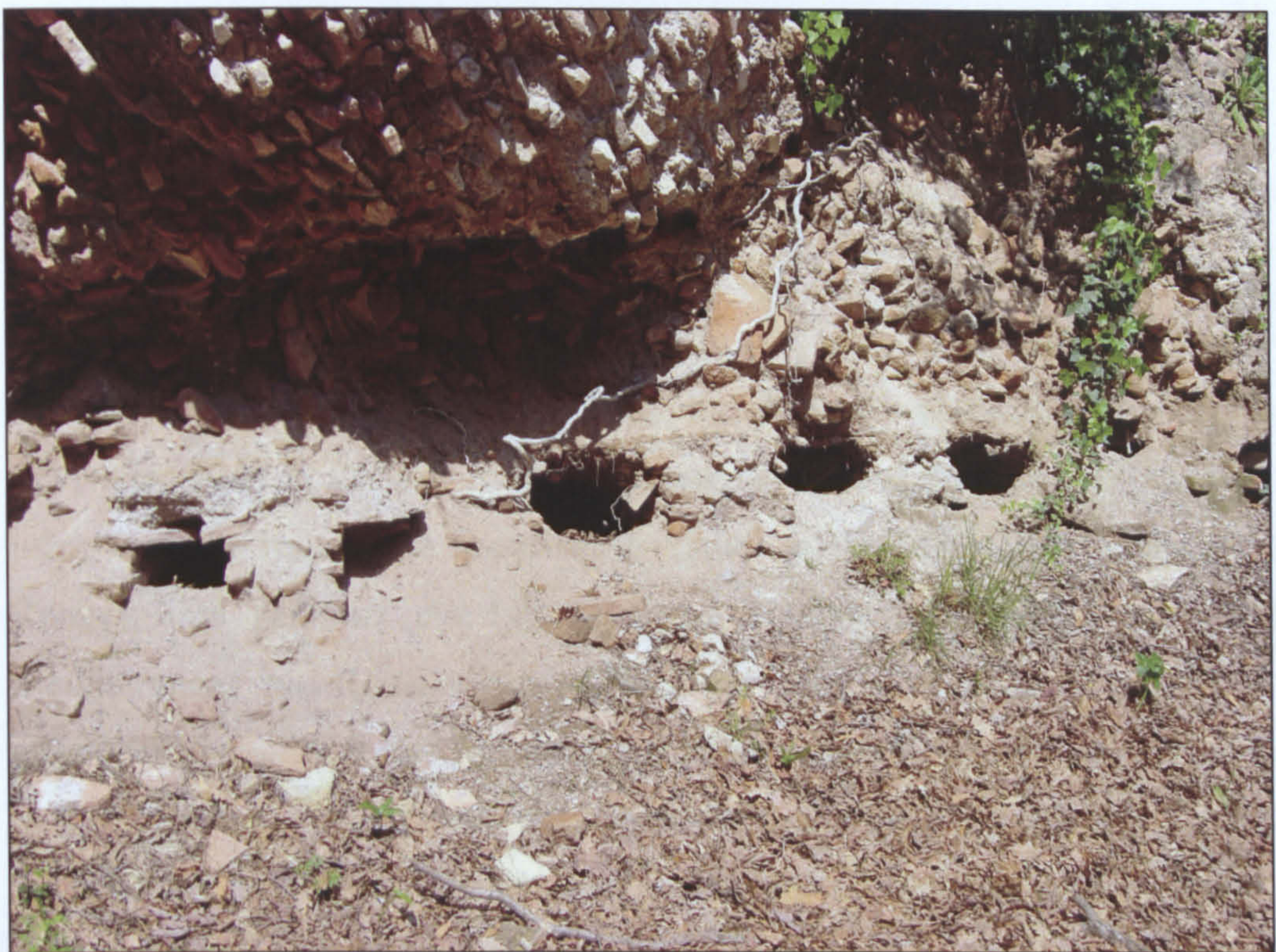
Fig. 3.15 Air vents underneath a granary store, Portus.
