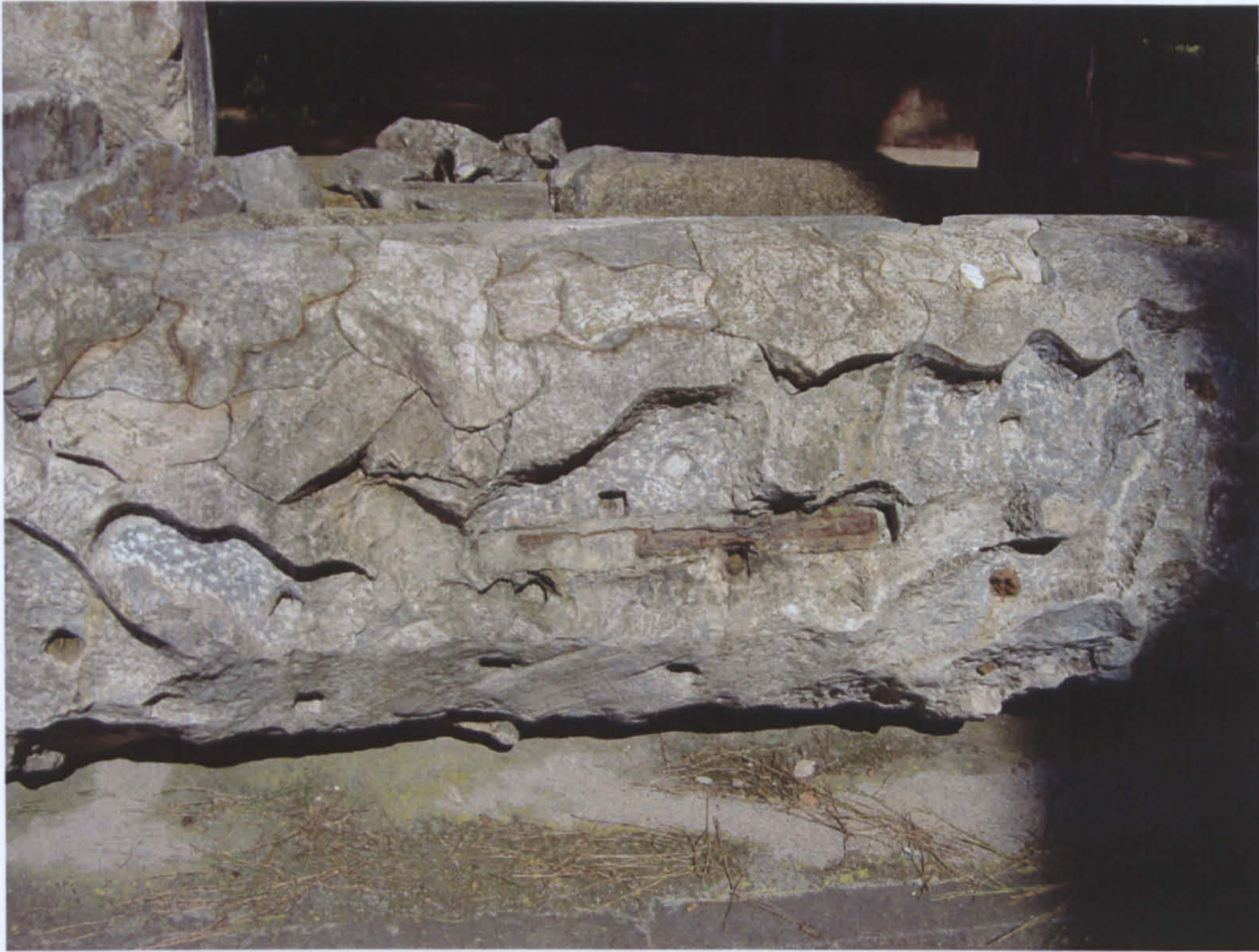
Fig. 6.15 Lead clamping in a block of marble from Portus.
