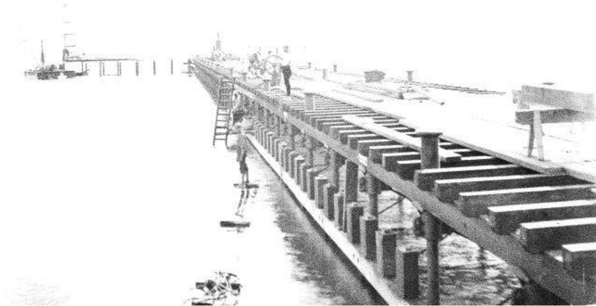
Figure 3.10 : Construction of wooden jetty at the harbour of Larnaka in the early 20th century (Marangou 1997 : 219). Photo taken by Coode & Partners.
