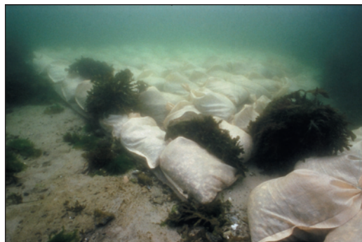
Figure 24.11: What is likely a short-lived attempt at stopping erosional destruction of the Nekselø fish weir. A small part of the feature is covered by fibertex and sand bags (Photo: Torben Malm)
