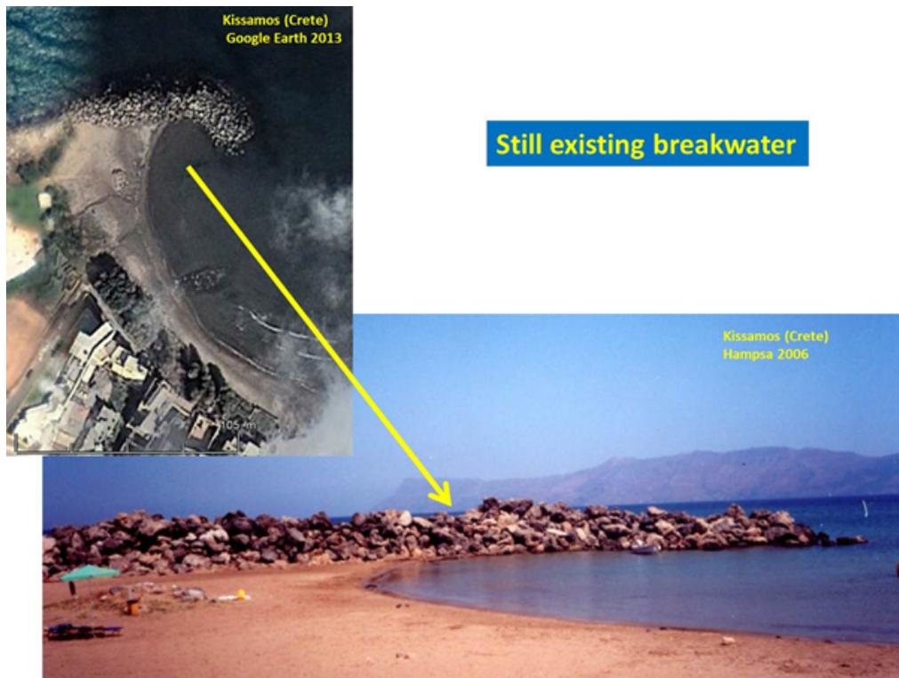
The Kissamos breakwater (Crete) is a typical example of a rubble mound breakwater. This particular structure has been preserved from wave attack due to tectonic uplift (Flemming, 1981). However, most ancient breakwaters were destroyed by wave action and their remains are found under water as “submerged breakwaters”.
