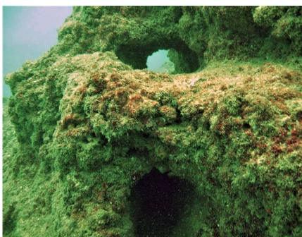
Belova's team in Alexandria<sup>139</sup>, reported a ca. 0.10 m hole near the edge of many large breakwater blocks (2 x 2 x 1 m). These holes have probably been used for ropes, either during construction of the structure, and/or for mooring ships later on.
