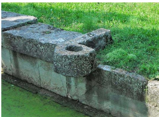
Possible foot-hole of a derrick mast at Aquileia
