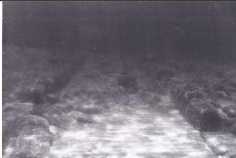
Between 'quay' 2 (right) & 3 (left), the dock is heavily sanded up and blocks from the top perimeter layer have fallen off. Pic. looking south, by Misson, 1965
