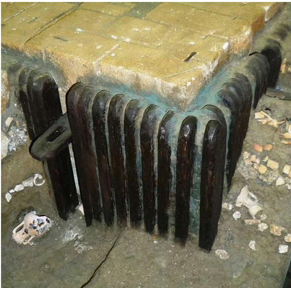
Detail of the model of the Môle de la Marseillaise at La Nautique near Narbonne (model built by Jean Marie Falguera). The piles are juxtaposed and tied by horizontal tie rods with a system of tenon and mortise that can still be seen. (Photo A. de Graauw, 2011)
