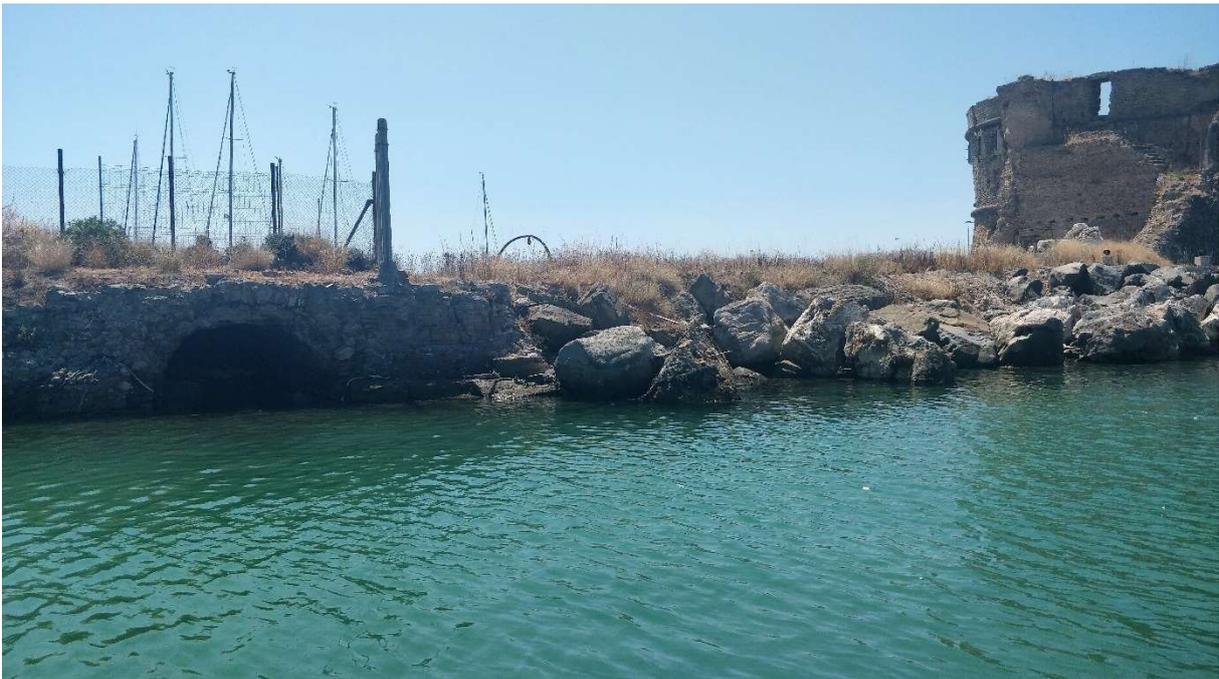
Molo del Lazzaretto, north side, open duct 4 and rock dumped in front of ducts 1, 2, 3 (photo A. de Graauw, 2022).
