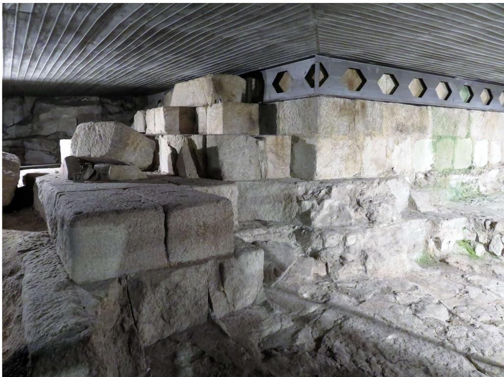
Tower of Hercules (A Coruna, Spain) showing reconstructed outer wall and ancient foundation level (A. de Graauw, 2017).
