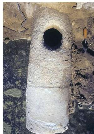
Fig. 9 – Mooring stone in grey granite from the S mole near Roman harbour entrance. The hole marks the probable setting of a timber crossbar and the unweathered lower part would have been embedded in the quayside.
