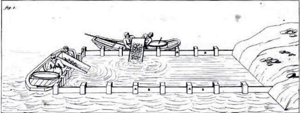
Claude Perrault's sketch (1673) with panels slid into grooves on poles, and labourers pouring concrete from the water surface which leads to segregation during the fall to the bottom.
