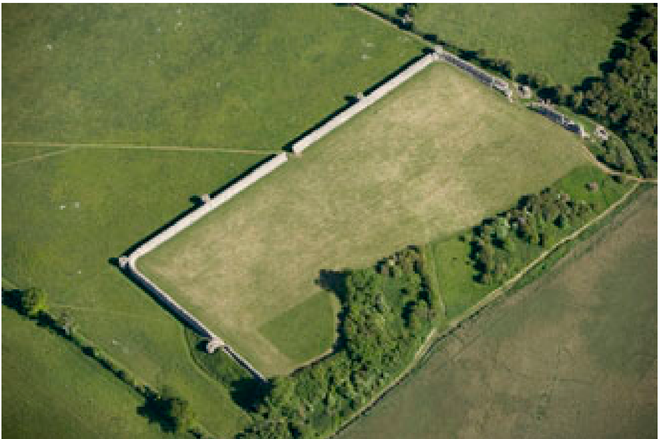
Figure 3 Aerial photograph of the bastioned fort at Burgh Castle, showing attrition (lower right) through coastal erosion.
