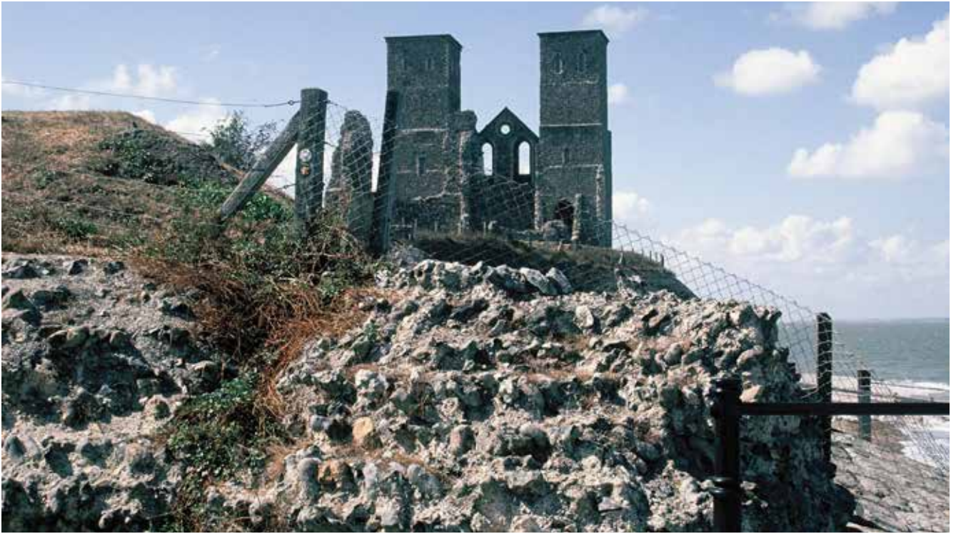
Figure 17 The towers of St Mary's church that were originally built at the centre of the Roman fort of Reculver but which are now perched on the cliff edge. Note the remains of the Roman walls in the foreground
