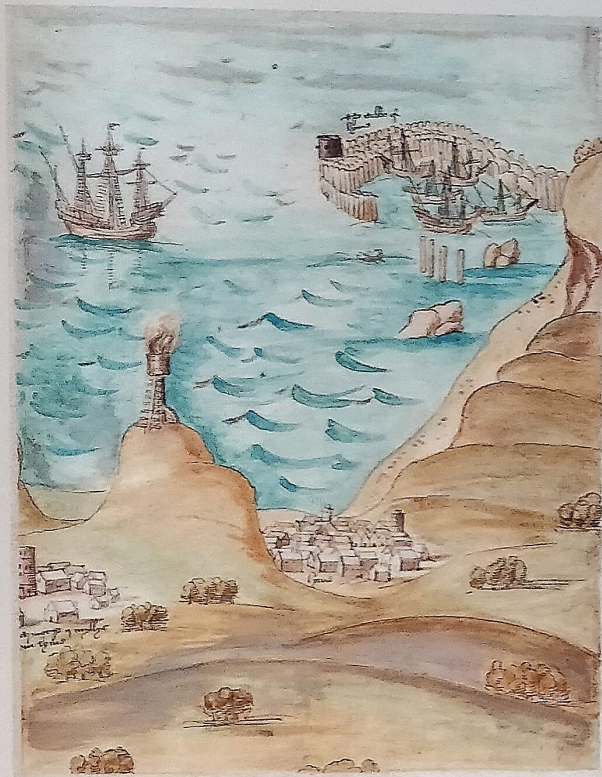
The earliest proper record of the Cobb is the drawing on a map made in 1539, showing it constructed of great banks of timber which enclose stone filling. The map is not very accurate, but does show a beacon east of Lyme, probably above Black Vein. By courtesy of the Dorset Museum.
