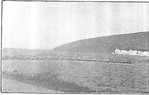
Figure 6. The Myrina Breakwater.
