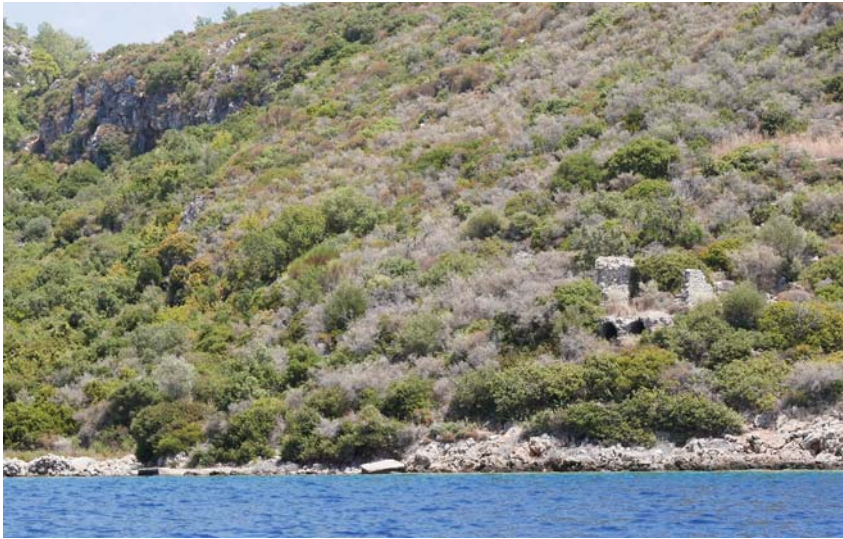
Fig. 10: Thyssanous, necropolis Area c: quay-like structure at shoreline (left) and Roman tomb building (right)
