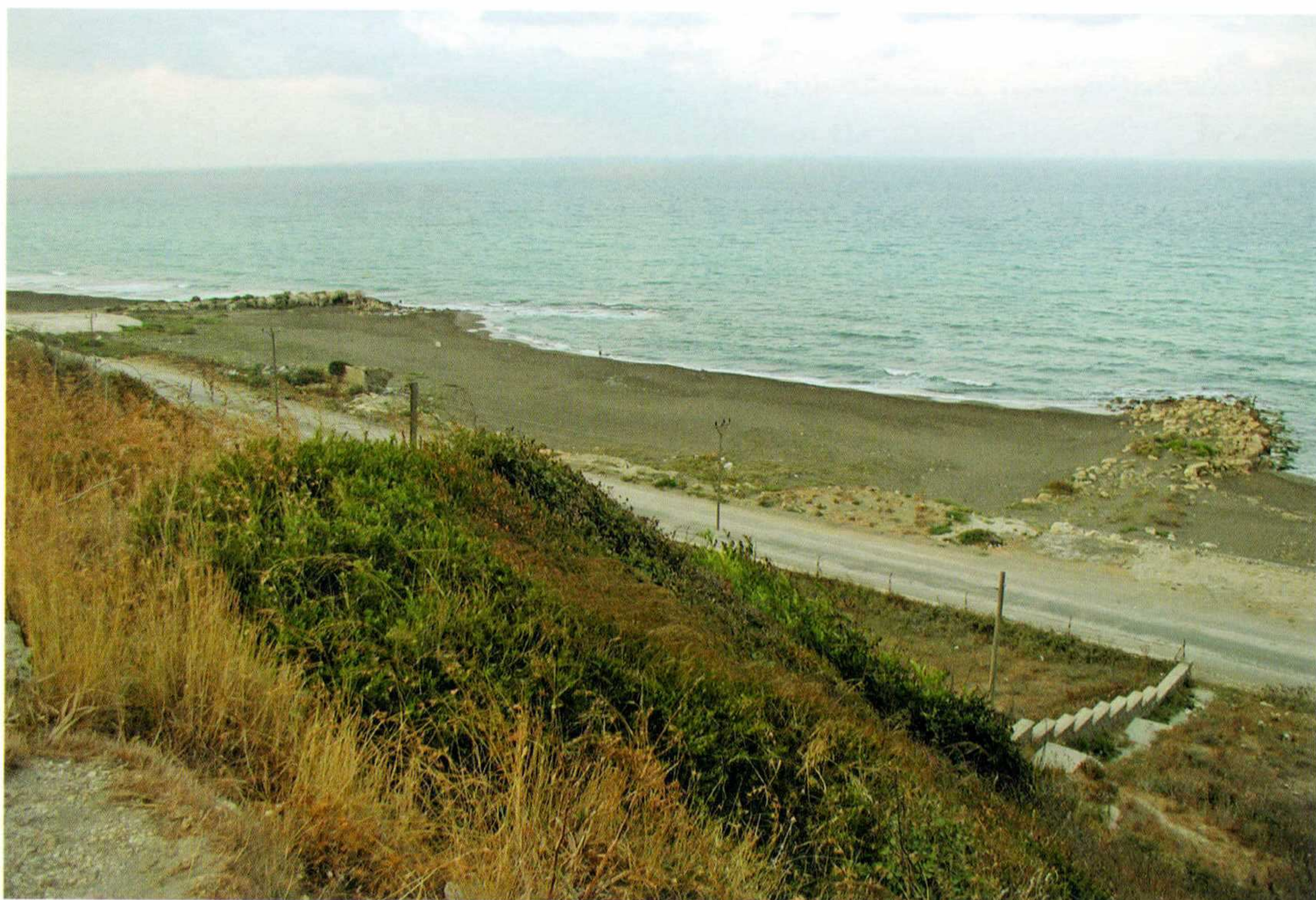
Fig. 28 General view of the exterior harbour from the east (ODAP Archive)
