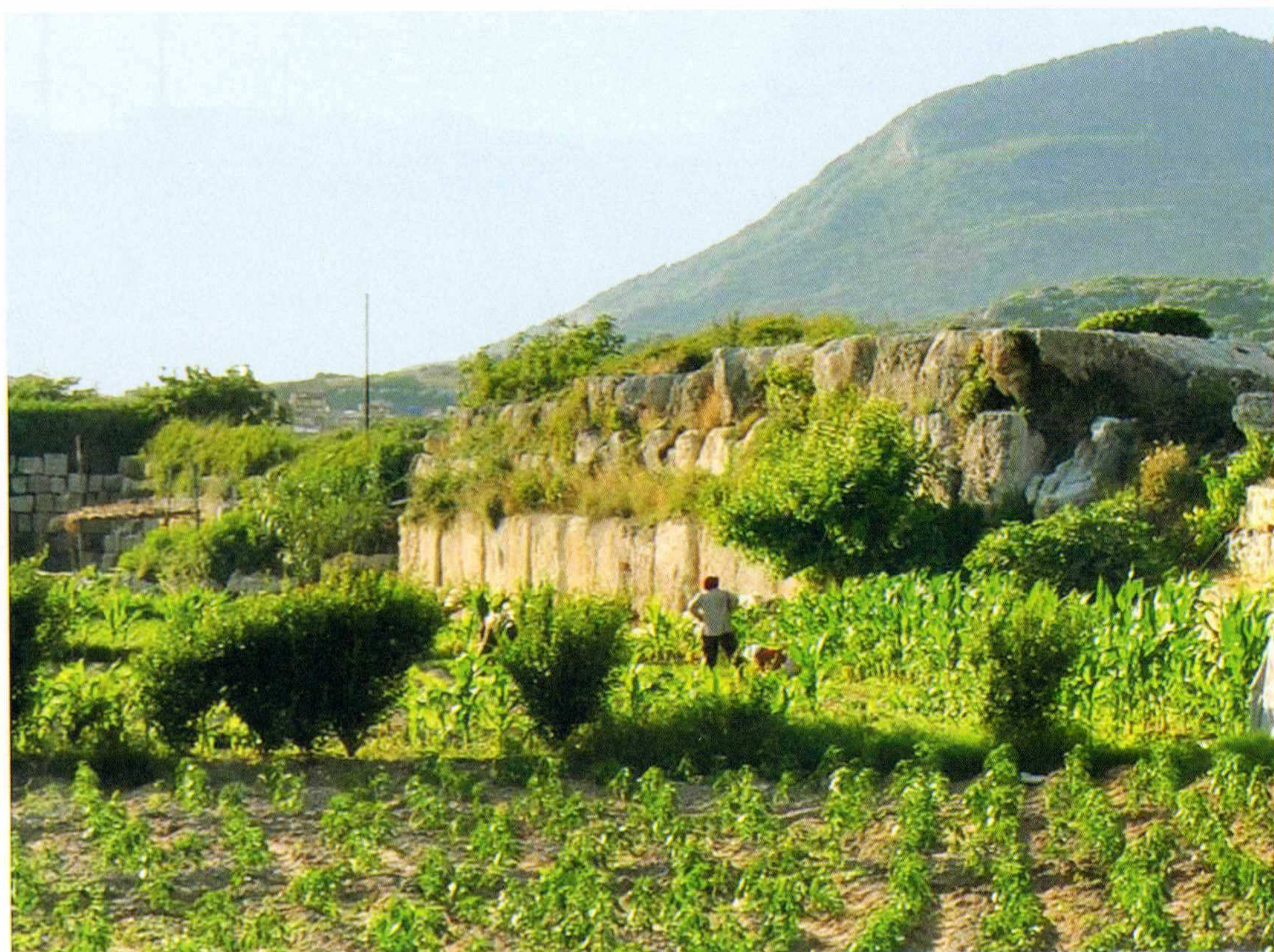
Fig. 10 North pier of the harbour (ODAP Archive)
