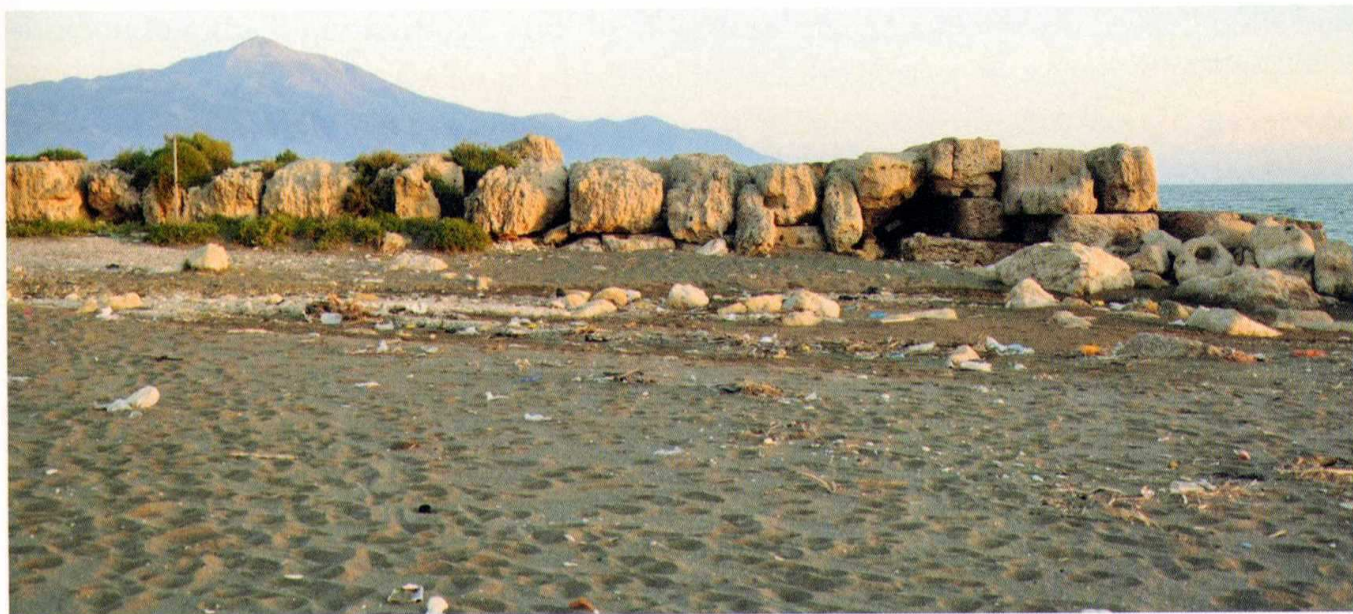
Fig. 26 Looking at the southern pier from the north (ODAP Archive)
