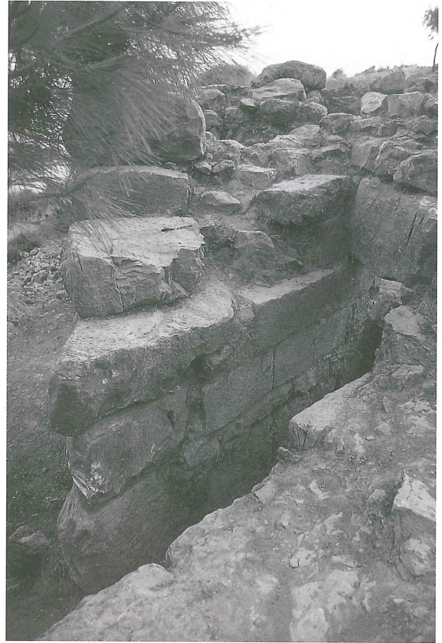
Res./Fig. 23 Kule 3 güney postern Southern postern at Tower 3
