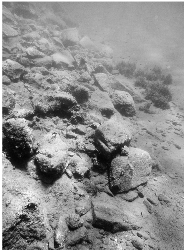
Figure 11. View of the exterior of the large rubble breakwater at the southern end of L4 (J. Leidwanger).
