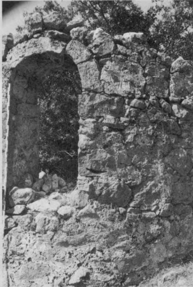
Photo 9: Karacaburnu, the church, main apse
