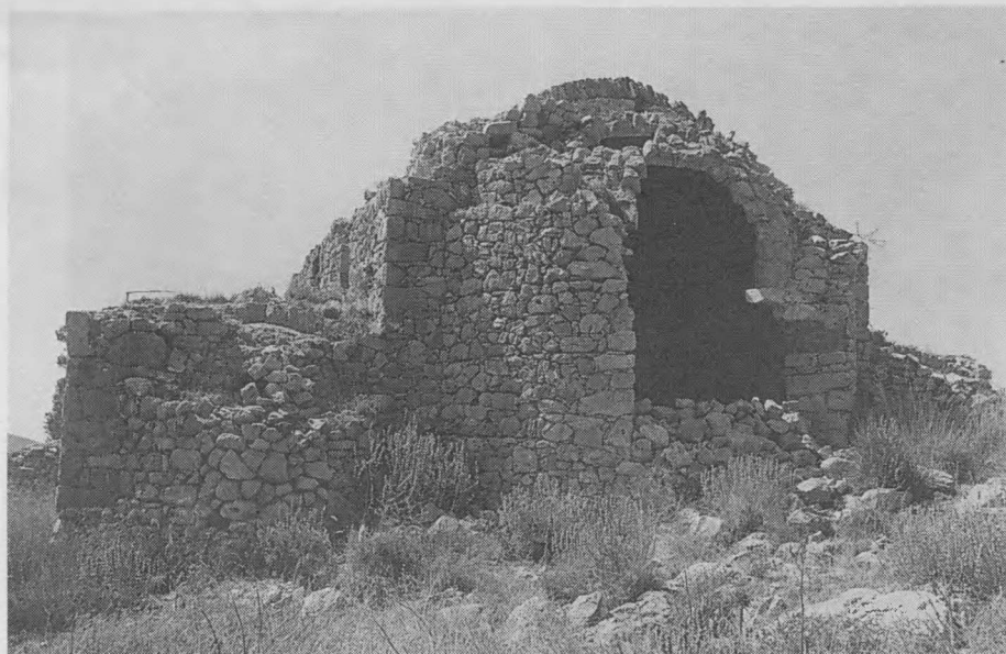
Photo 8: Tavşan Adası, the church from east
