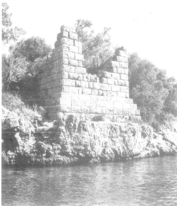
Fig. 3. — Kedrai, bastion monumental.
