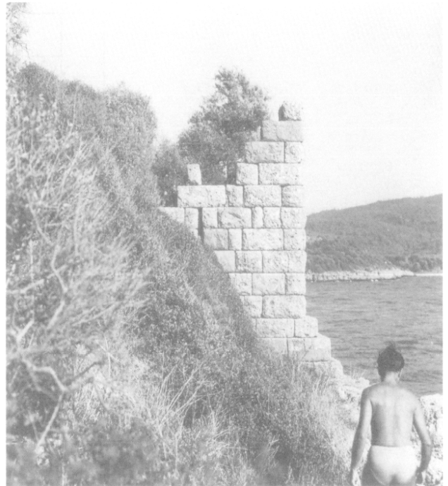
Fig. 2. — Kedrai, bastion monumental.
