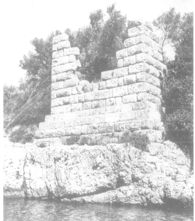
Fig. 4. — Kedrai, bastion monumental.
