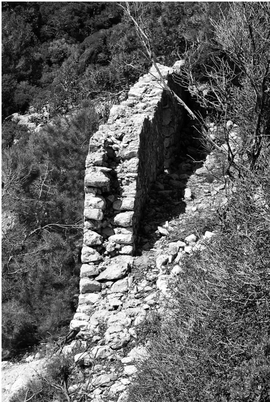
Fig. 38 Gavur Kalesi. Detail of the masonry
