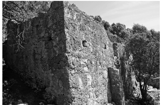
Fig. 39 Gavur Kalesi. Detail of the masonry
