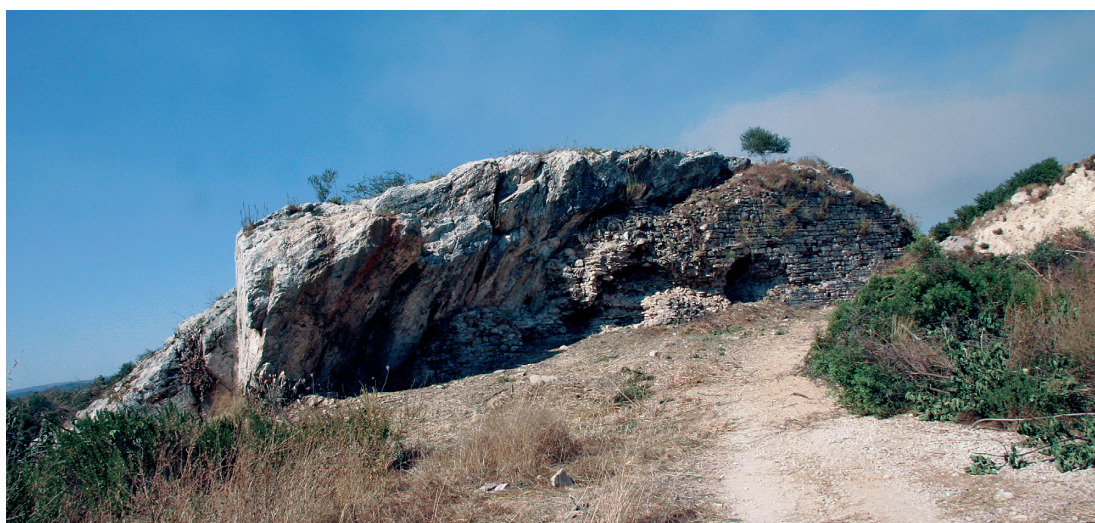
Fig. 13 Roman building on the Çanakgöl Tepe in Ephesos (M. Steskal © OEAI)
