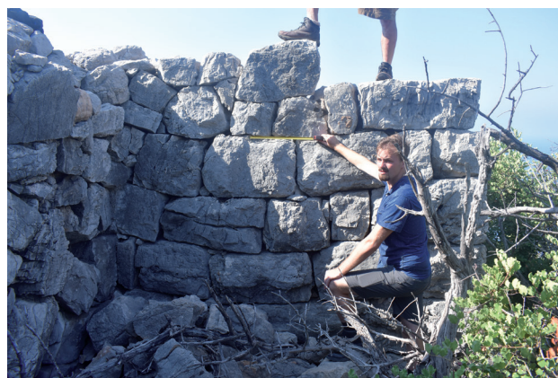
Fig. 17: View of North Face of Tower on South Wall, Aphrodisias
