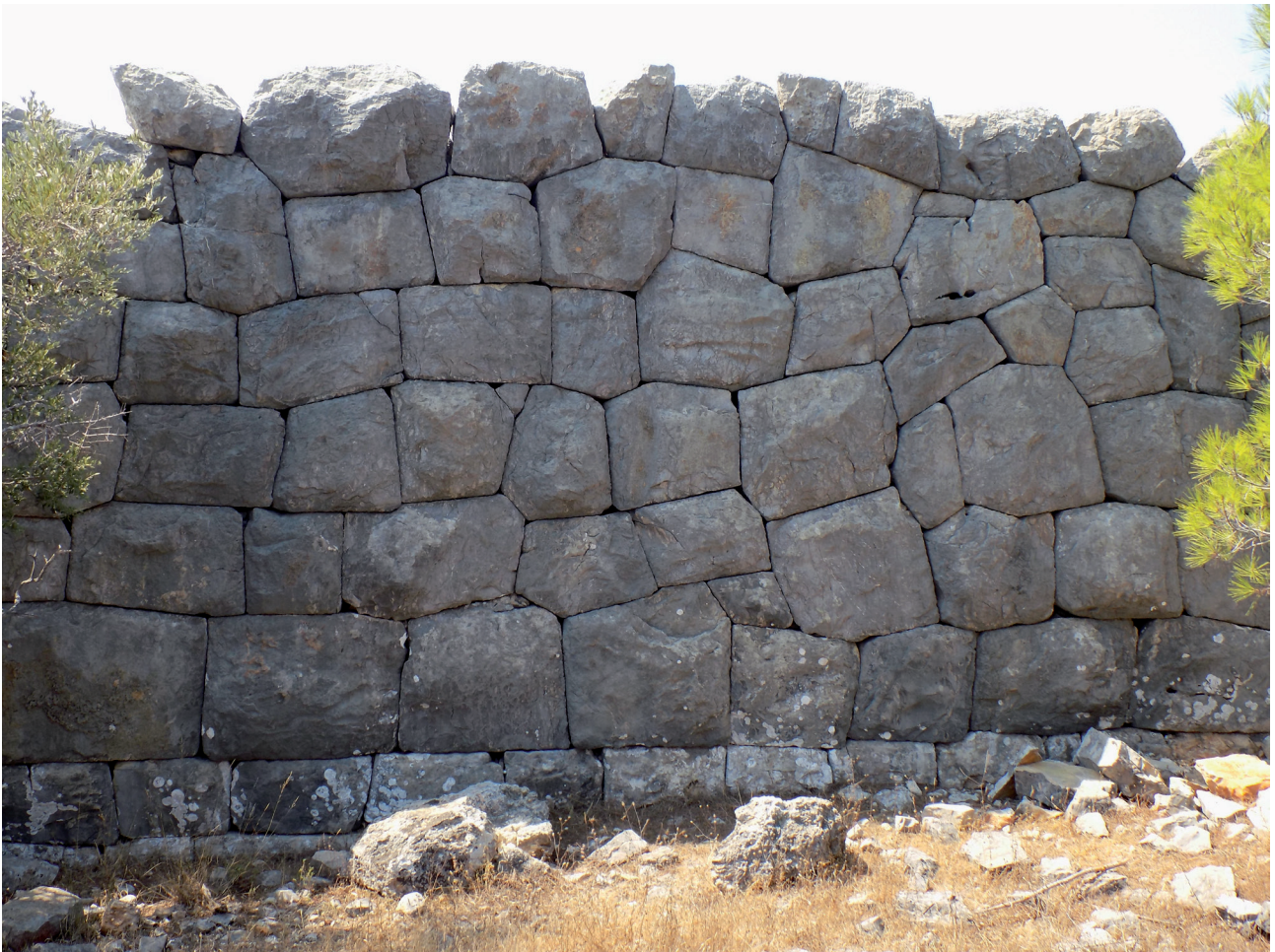
Fig. 14: Polygonal Masonry Technique, Interior Face of Platform Adjoining Tower 15
