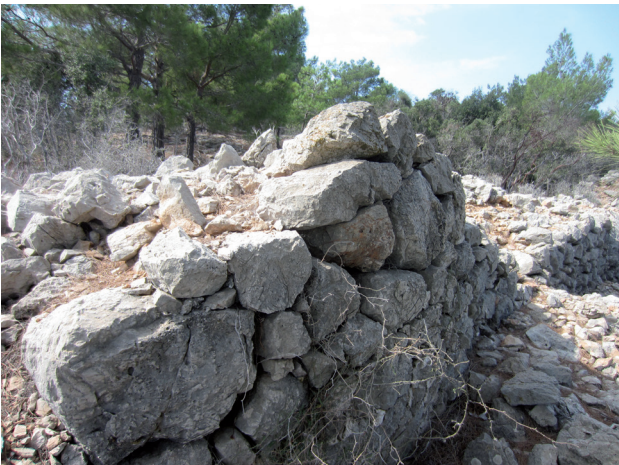
Fig. 5: Southeast face of Dana Kale One (Phase 1)
