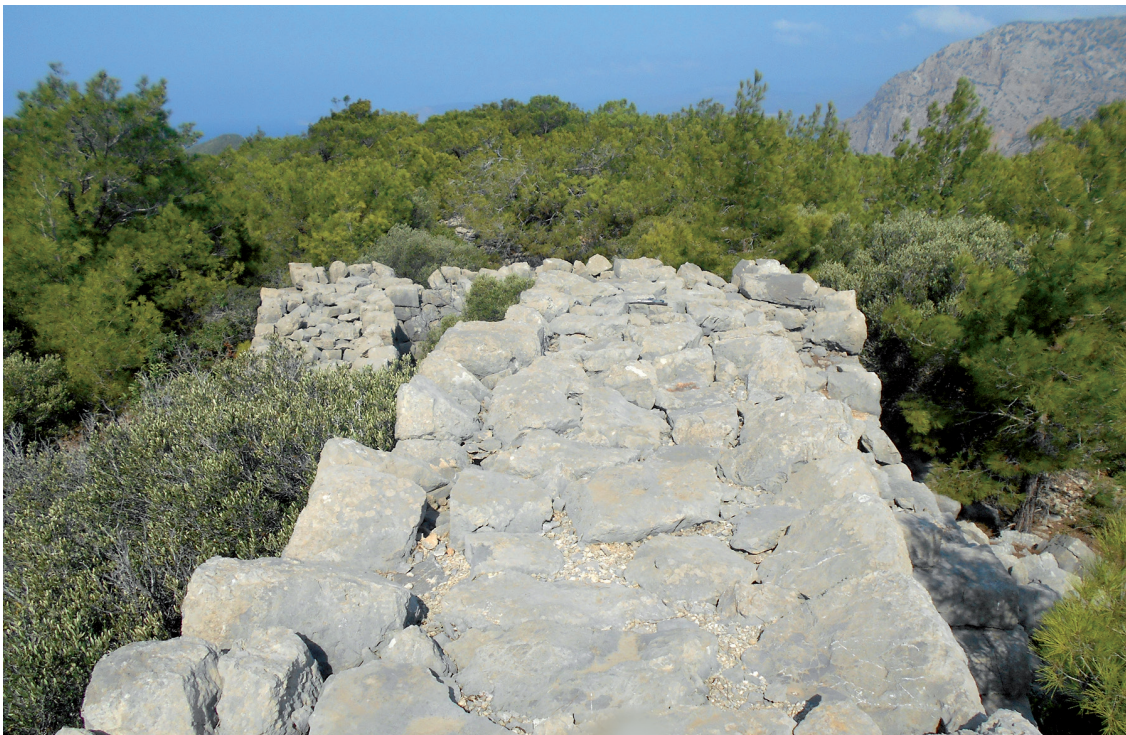
Fig. 12: View of Platform at Tower 15 (Remains of Tower in Foreground, Remains of Stairway to the Right), Aphrodisias North Wall
