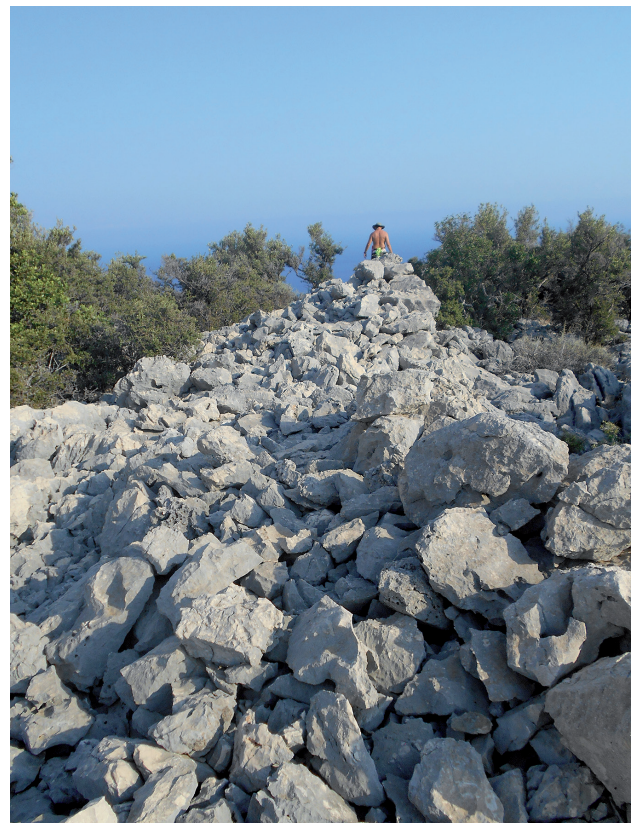
Fig. 10: Wall of Pentagonal Fortress on north flank of Tahta Limanı
