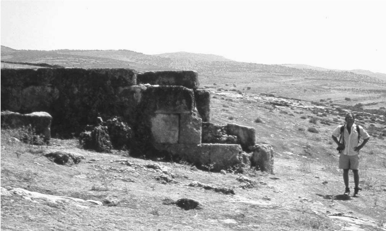
Figure 2.28. Masonry Penstock of a Roman/Late Roman Water Mill at Khirbet al-Tahoun (AS 171), Looking Southeast
