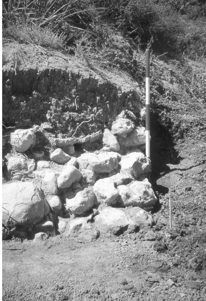
Figure 2.7. Close-up of the Roman Building Shown in Figure 2.6, Showing Stones and Overlying Roof Tiles
