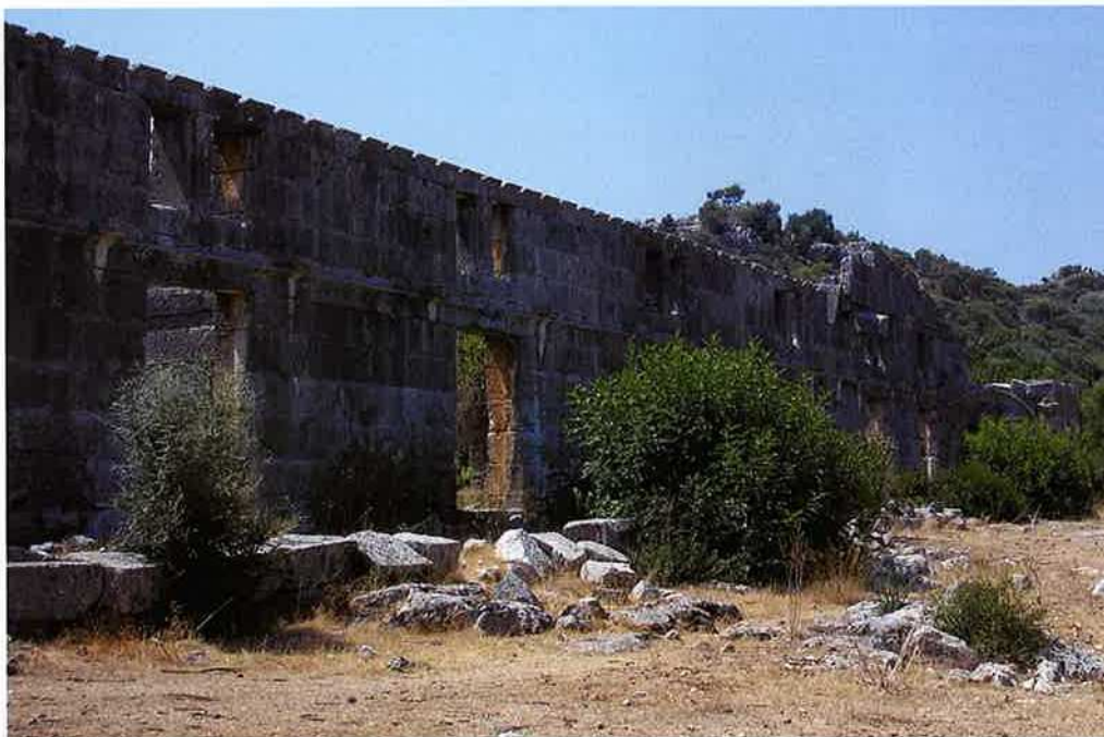
The large horrea at Andriake. Built to store grain in eight separate rooms, the early 2nd century building is remarkably well preserved. Photo: James Beresford.
