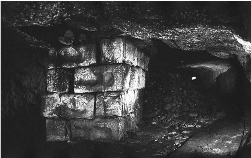
Fig. 5: Galeria do Pilar. Looking north from behind the pillar towards the entrance. Around the pillar the gallery was enlarged towards the East. The channel is visible in the enlargement. The pillar consists of 24 mortars (Photo: C. Wahl).
