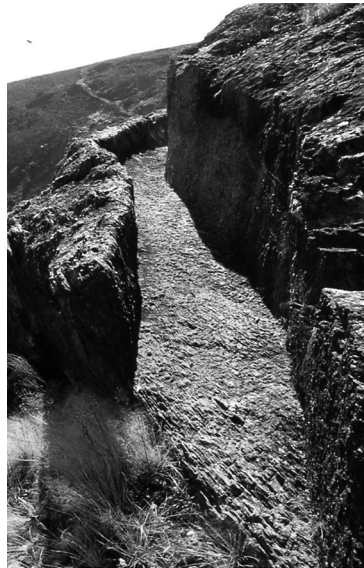
Fig. 2: Aqueduct cut into the rocks, seen from the North (Photo: J. Wahl).
