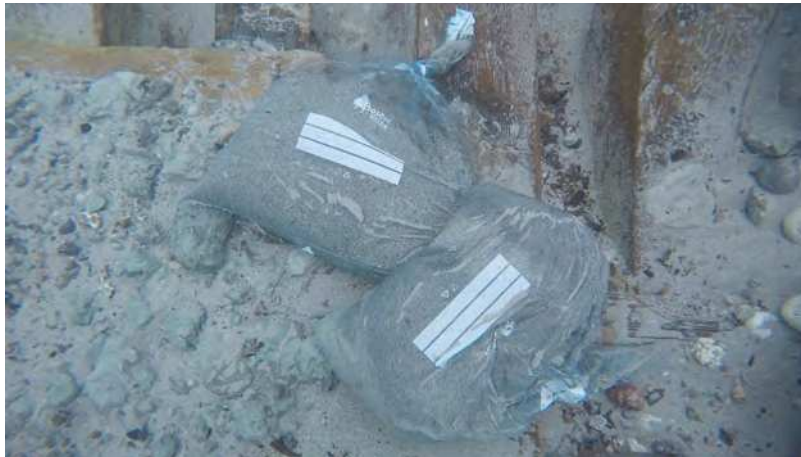
Figure 7. Use of sand bags for the consolidation system.
