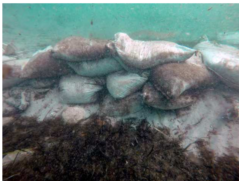
Figure 12. Retaining wall with sand bags reused for physical protection in situ, where the effectiveness in stopping the entry of dead posidonia is observed
