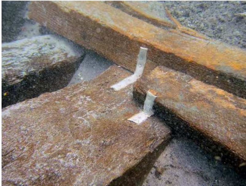
Figure 6. Photograph of consolidation with polyester resin strips.
