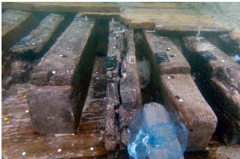
Figure 8. Use of sand bags for the immobilisation of structural parts.
