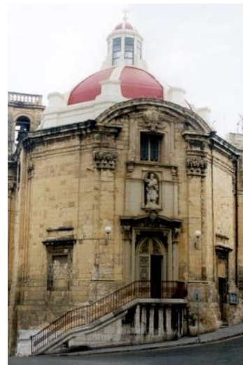
Fig. 3. The lower part of the church façade shows the white limewashes applied before 2010.
