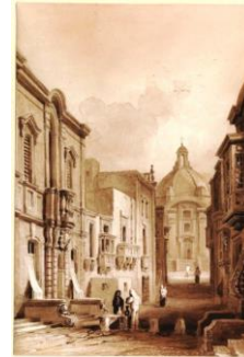
Fig. 5. A drawing by Owen Browne Carter (1829) showing St. Paul's Street and Church at Bormla, Malta.
