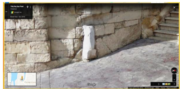
Fig. 2. The cross-column uncovered in 2010 is inserted between the rocks and the foundation blocks of the church. Picture: Courtesy of Google Maps street view.
