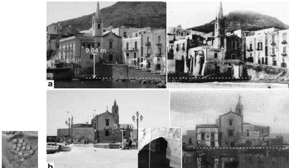
Fig.10: a) View of S. Giuseppe church (site 2-e); how it was at the beginning of the XX century and how it appears at present. b) View of the church Anime del Purgatorio (site 2-d); how it was in August, 1913 and how it appears at present; in the inset note the ground floor partially submerged. Both pairs of pictures are taken from the same perspective and the scaled together. The red lines indicate the common recognizable features and the dashed yellow lines refer to the present-day average sea level.
