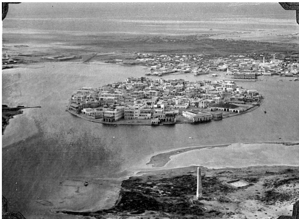
Figure 2. Aerial photograph of Suakin in 1930 (Durham University, Sudan Archive). Since this photograph was taken the condition of the buildings on the island has deteriorated considerably and most have now collapsed.
