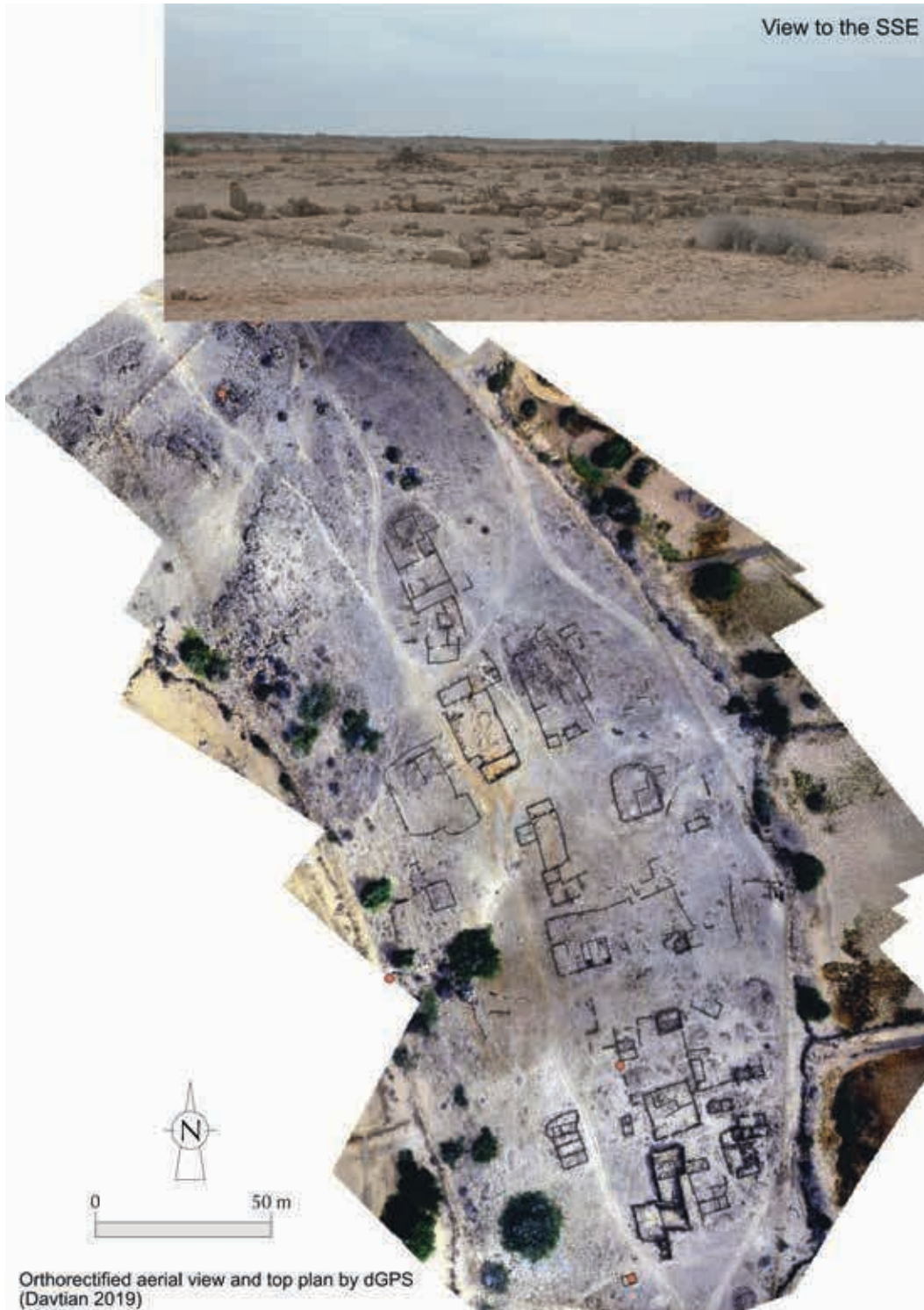
Fig. 11 – Aerial orthorectified view and top plan of the remains in Ġurayn and view of the remains to the southeast (orthophoto: G. Davtian 2019; photo: S. Marion de Procé/MIFA 2019).
