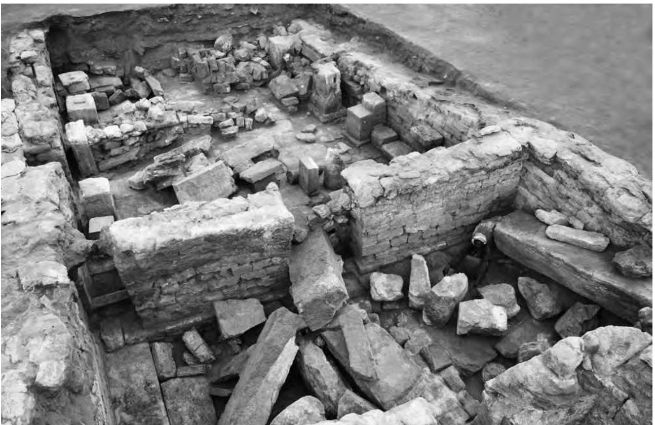
2: Isis Temple (not including the propylon area). Area with sandbags to extreme left is trench BE19-122. View looking east southeast (photo by S.E. Sidebotham)
