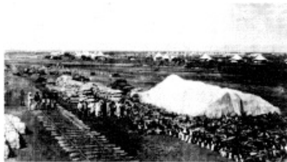
Figure 2.5 A photograph showing the construction of the railway and the British camp (from Myatt 1970)
