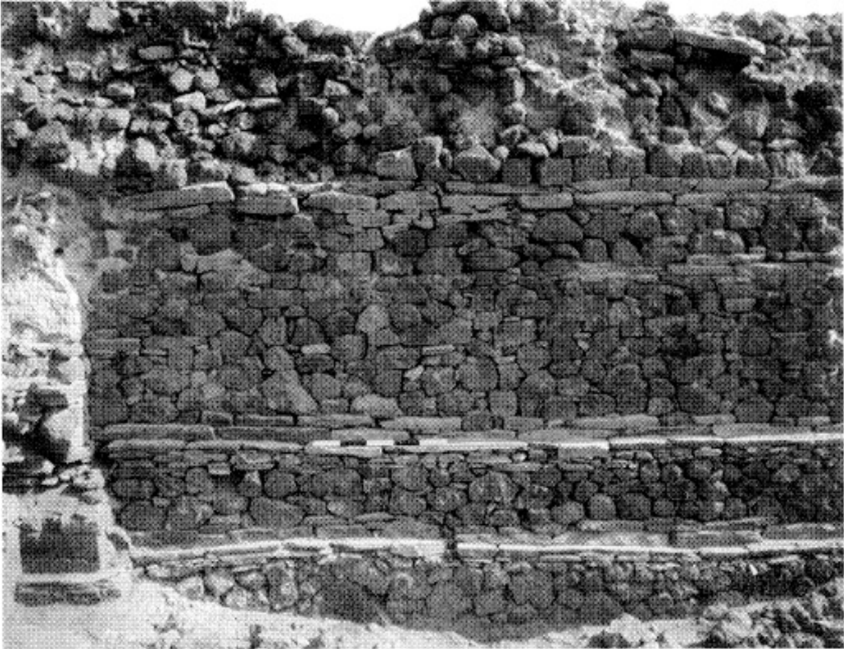
Figure 9.2 View of the main wall exposed in Anfray's trench
