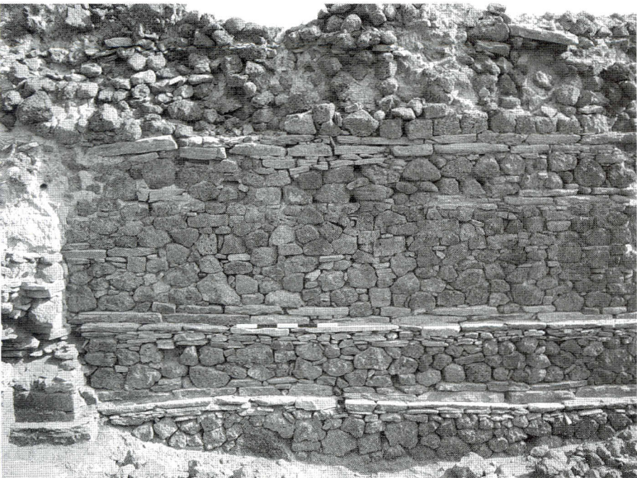
Figure 9.2 View of the main wall exposed in Anfray's trench
