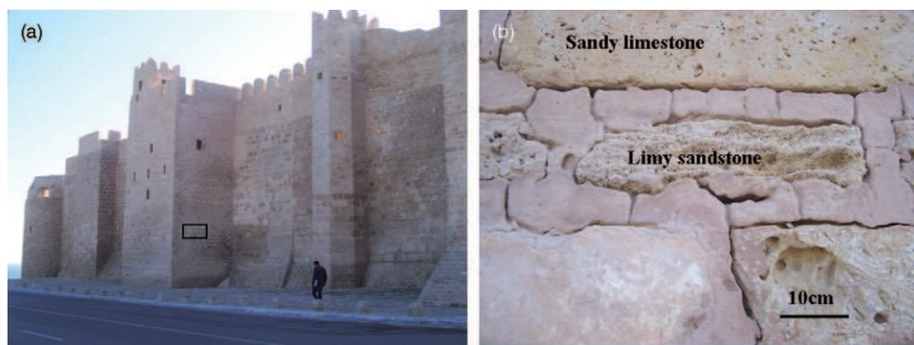
Figure 10 A panoramic view of the Ribat (a) and a detail of the wall (b).
