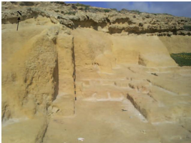
Figure 4 Quarry 1: marks of extracted blocks left on the quarry face.
