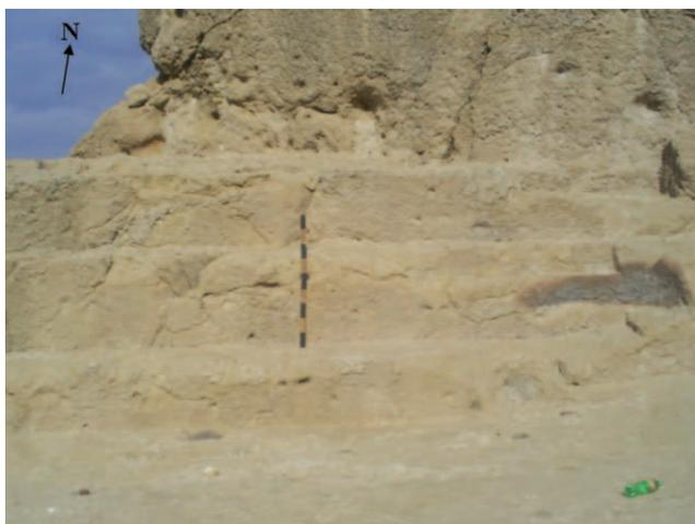
Figure 5 Quarry 2: part of the northern face of the quarry, showing three levels left on the quarry face after the extraction of blocks.
