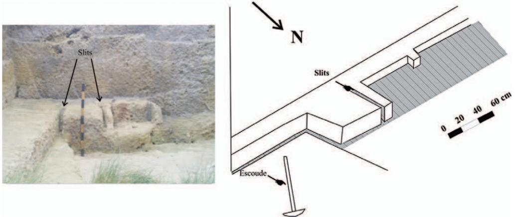
Figure 7 Quarry 4: part of the southern face of the quarry, showing marks of extracted blocks left on the quarry face. A pre-cut block can be seen in the foreground, with an extracted one just to its side.
