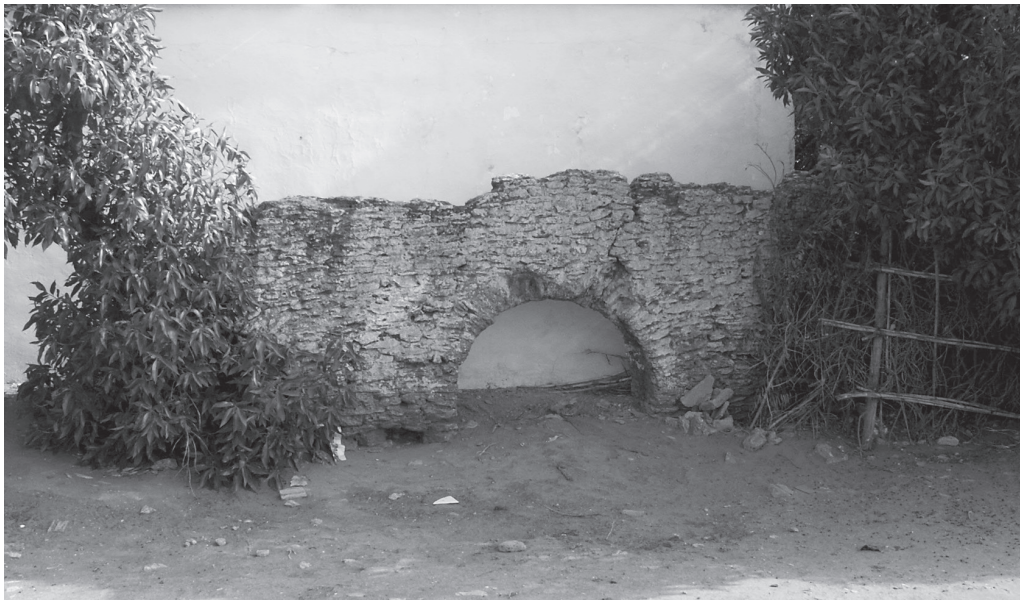
FIG. 82. PART OF THE AQUEDUCT ON THE BLUFF, BUILT INTO A HOUSE, 2002. APPROXIMATELY 1 M HIGH (PHOTO: AT).
