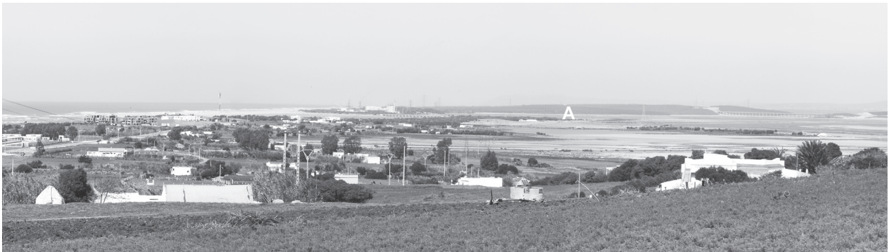
FIG. 53. OVERVIEW NORTH TO THE FISH-SALTING COMPLEXES AT TAHADART (A), SITUATED ON THE WESTERN EDGE OF THE LAGOON FORMED BY THE OUEDS TAHADART AND HACHEF, 2007. THE ATLANTIC IS TO THE LEFT (PHOTO: AT).
