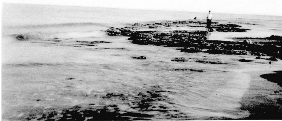
2. Looking seaward along the sea leg of the breakwater
